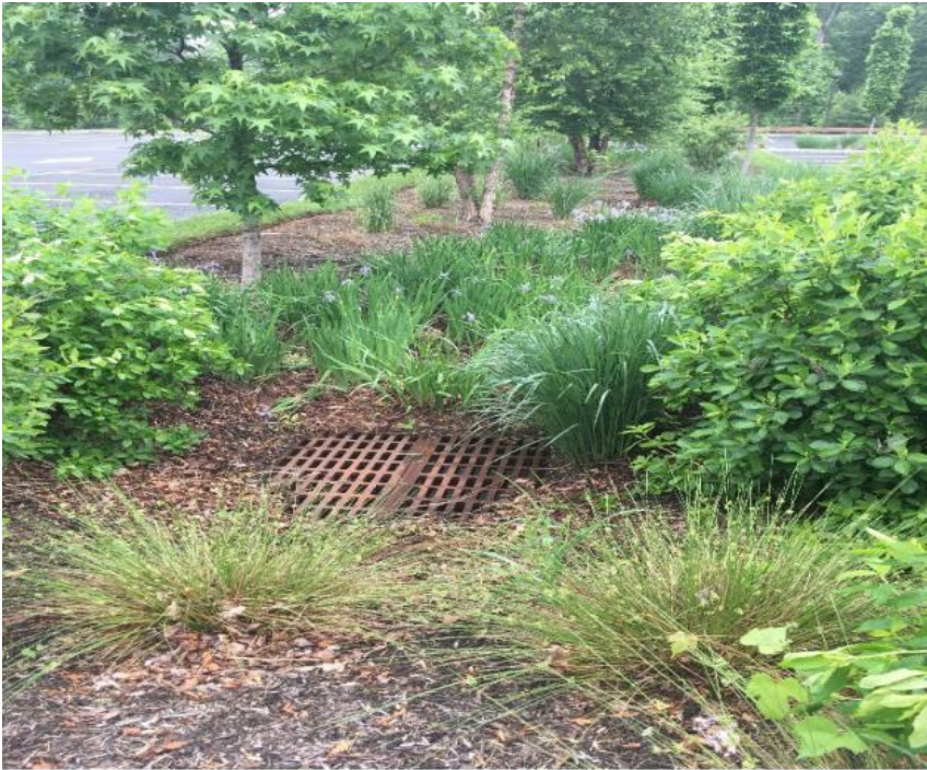
Bioretention center parking aisle, Princeton, NJ
