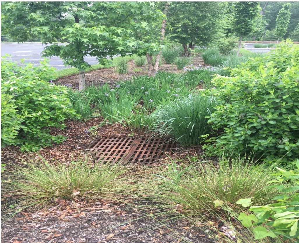
Bioretention center parking aisle, Princeton, NJ Photo by DEP Stormwater Engineer Lisa Schaefer
