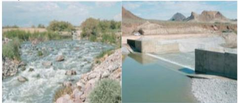
Weirs are low dams designed to reduce streambed erosion by flattening the slope of the channel and slowing flows. Many weirs are constructed of confined rock riprap, providing a somewhat natural look (top). Other structures are built with concrete, resulting in a more engineered look (bottom). Weirs, wetland restoration, and invasive vegetation removal helped reduce total suspended solids (TSS) concentrations in lower Las Vegas Wash and led to its removal from the Nevada 303(d) list in 2004.
