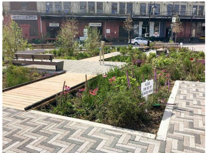
Hoboken City Clean Water Project, Southwest Park & Underground Retention System
