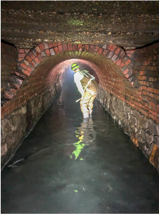
Camden County Municipal Utilities Authority Clean Water Project
