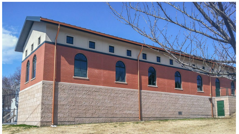
Milltown Borough Electrical Substation Relocation
