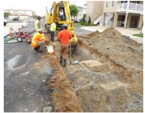
North Wildwood Sewer, Storm and Street Restoration
