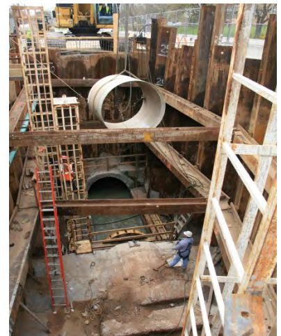
Passaic Valley Sewerage Commission Interceptor Slip Lining
