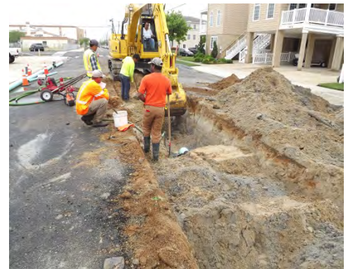
North Wildwood Sewer, Storm and Street Restoration
