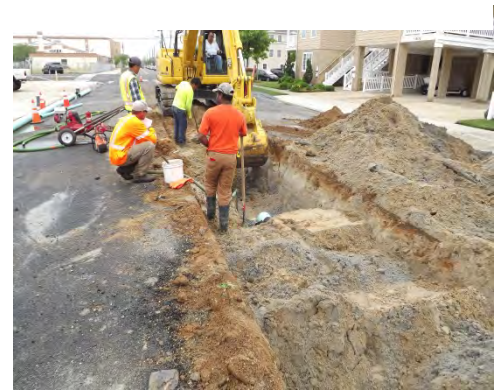
North Wildwood Sewer, Storm and Street Restoration
