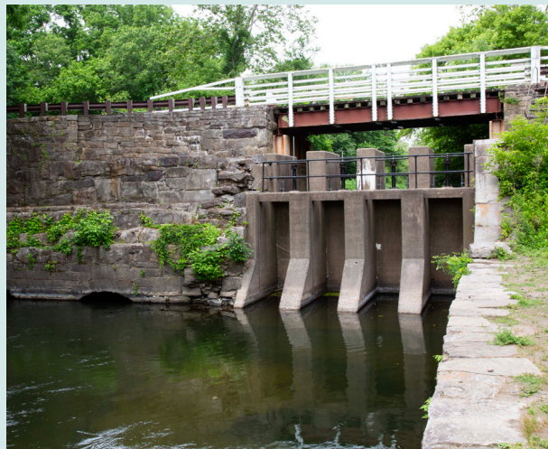
Guard Lock on Delaware and Raritan Canal in Bulls Island State Park near Stockton.
