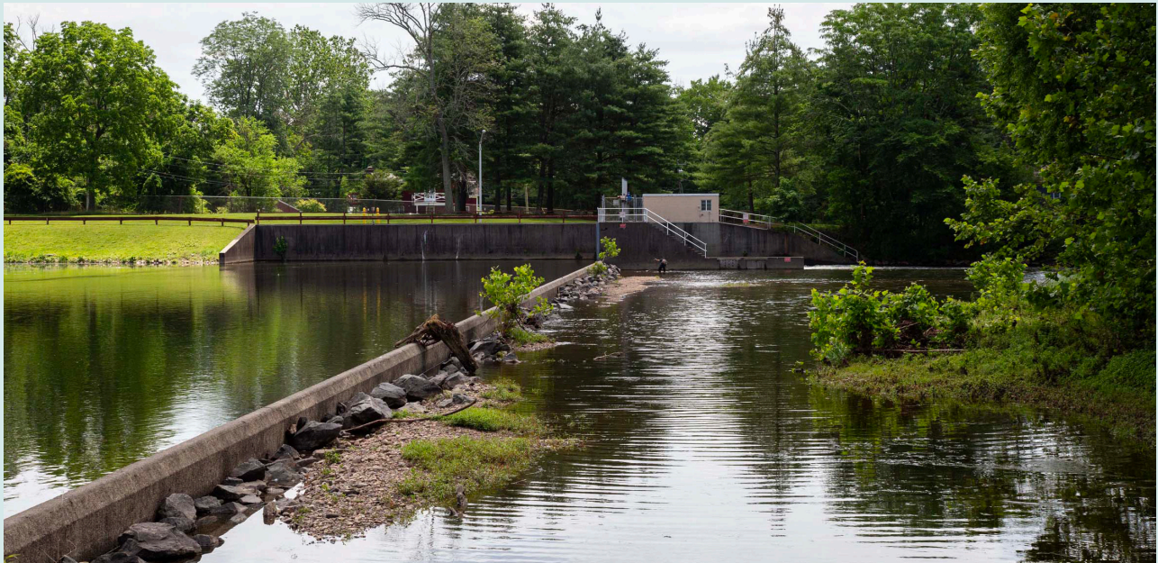
Hamden Pump Station operated by the New Jersey Water Supply Authority in Clinton Township, New Jersey. This station allows water to be moved from the Raritan River into Round Valley Reservoir.
