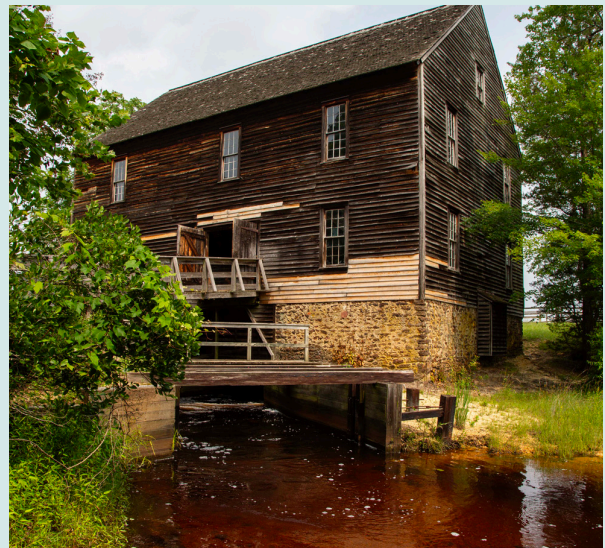
Batsto Village located in the Wharton State Forest in the Pinelands National Reserve. The tea-color water is a natural characteristic of the streams in the New Jersey Pine Barrens.
