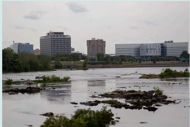
Delaware River looking downstream from the Calhoun Street Bridge in Trenton. This historic bridge crosses the Delaware River, connecting Trenton, New Jersey with Morrisville, Pennsylvania.
