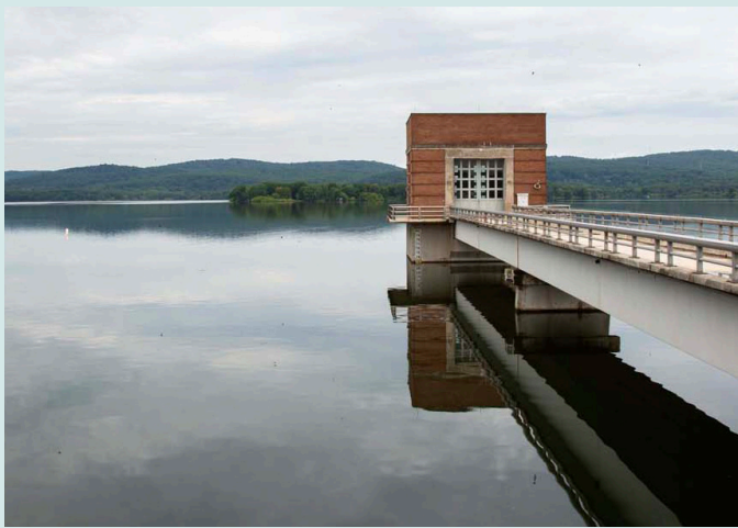
A water release at Spruce Run Reservoir in Clinton, New Jersey. This reservoir is considered one of the first water supply facilities to be constructed and operated by the state.
