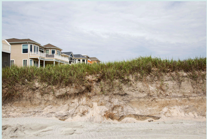
A revetment and shorefront community located in Brigantine, New Jersey. Sea level rise poses a risk to critical infrastructure and water resources located in New Jersey's coastal areas.
