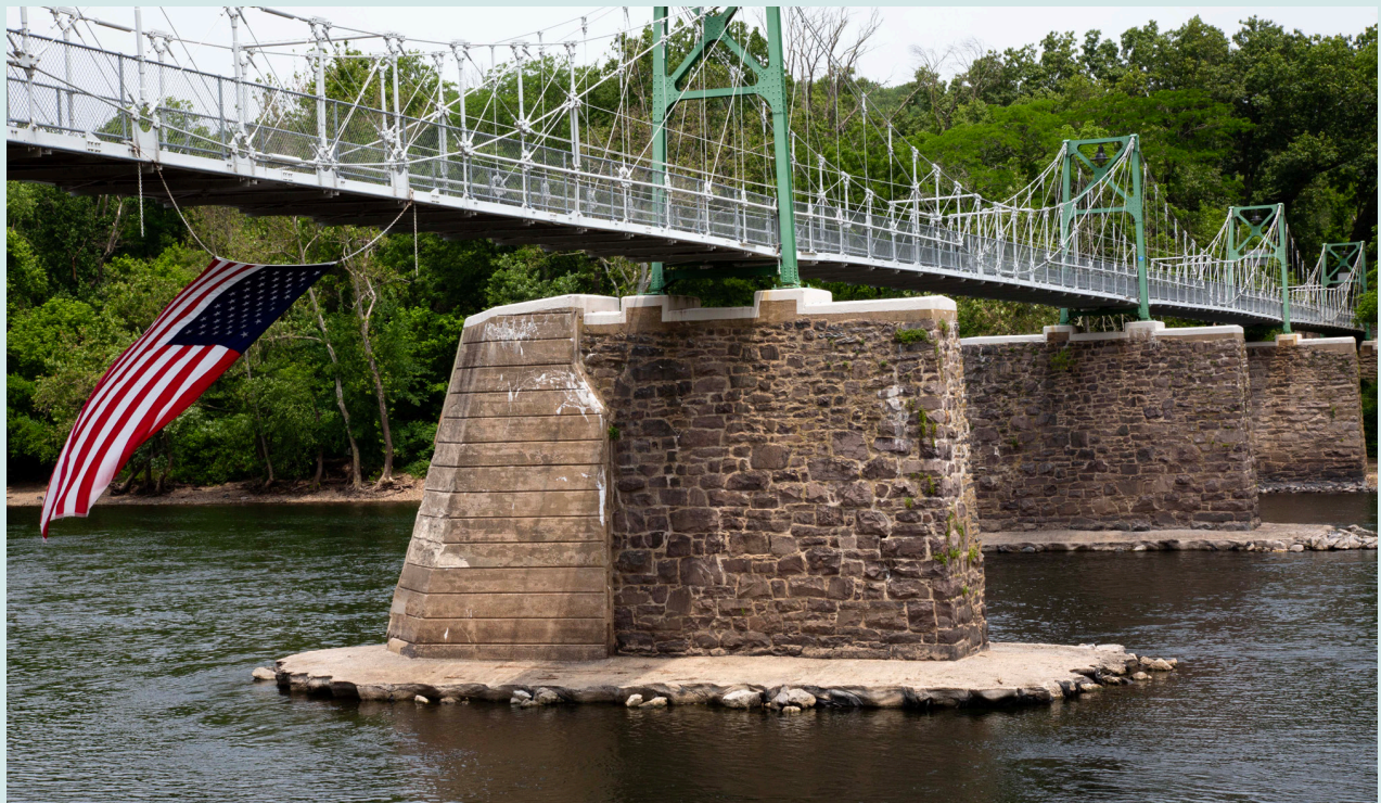
Pedestrian Bridge over Delaware River at Bulls Island Recreation Area, Stockton NJ.
