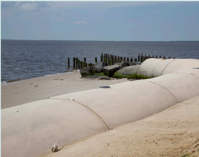
Beach erosion control structure near East Point in Cape May County.
