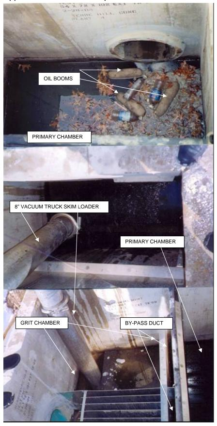
The Primary Chamber is where the stormwater enters. The water may enter through pipes or an inlet grate in the lid.
