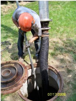
A maintenance worker stationed on the surface uses a vacuum hose to evacuate water, sediment, and debris from the system.
