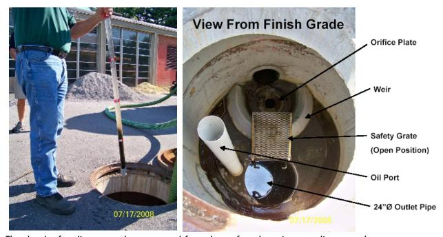
The depth of sediment can be measured from the surface by using a sediment probe or dipstick tube equipped with a ball check valve and inserted through the 24-inch outlet riser pipe. Oil level can similarly be checked through the oil inspection port.
