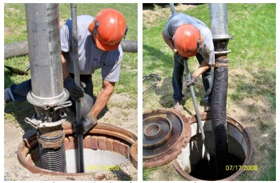
A maintenance worker stationed on the surface uses a vacuum hose to evacuate water, sediment, and debris from the system.
