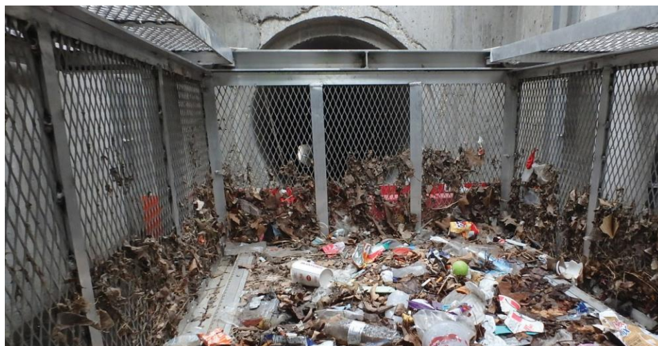
Nutrient Separating Baffle Box with collected trash, organics and debris inside the screened basket system ready for disposal.
