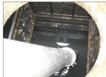
Open lower screen panels to remove sediments via vacuum truck.
