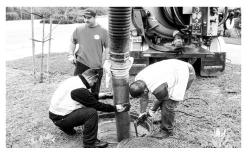
1. Remove access hatches set up vacuum truck to clean the pretreatment chamber.
