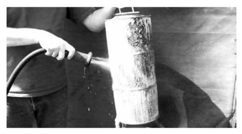
4. To wash cartridges, remove from vault. Place over trash can and use a garden hose to spray clean.
