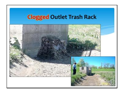
These two photos show a detention basin with a low flow channel. The trash rack to protect the low flow orifice is entirely clogged by debris and vegetation. The easy solution is to remove the debris and vegetation, but it may be necessary to conduct more frequent inspections and perform preventive actions to keep the trash racks clear.
