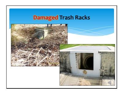
These two photos show the trash racks of a detention basin that has been damaged. Corrective action is necessary to affix the trash racks onto the outlet structures. More frequent inspections may be necessary to check if it has fallen off entirely.
