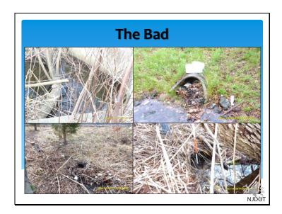
However, it is not always sunny here in New Jersey; it has to rain sometime. Here are a few examples of inlets in bad condition. These can be easily fixed by clearing the sediment, trash and vegetation. However, the quick fix will not be the best way to keep these bad conditions from re-occurring. We need a long term, consistent way to prevent these bad situations.
