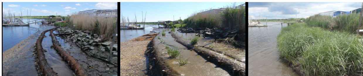
Fig. 11. Living shoreline installation in Delaware Bay, NJ. Initial installation (left panel) stabilized by coir logs and rock sill (middle panel) leading to subsequent revegetation with Spartina alterniflora (cord grass) (right panel). Image courtesy of Living Shorelines in the Delaware Estuary 2012.
