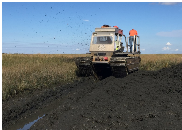
Figure 7. Runnel installation at Cape May NWR. Image courtesy Wood.
