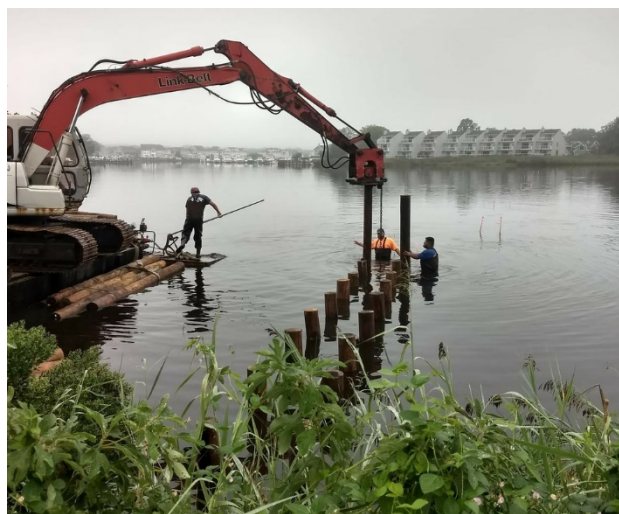
Fig. 14. Installation of wooden pilings to hold recycled Christmas trees. Image courtesy of American Littoral Society.
