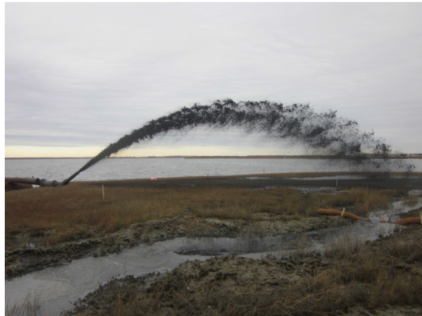
Fig. 4. Dredge sediment placement via a spray nozzle. Image courtesy NJDEP.
