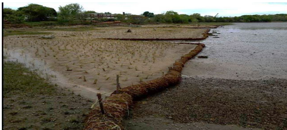
Fig. 12. Example of marsh creation with coir log toe protection. Image courtesy of Living Shorelines in New England: State of the Practice. 2017.
