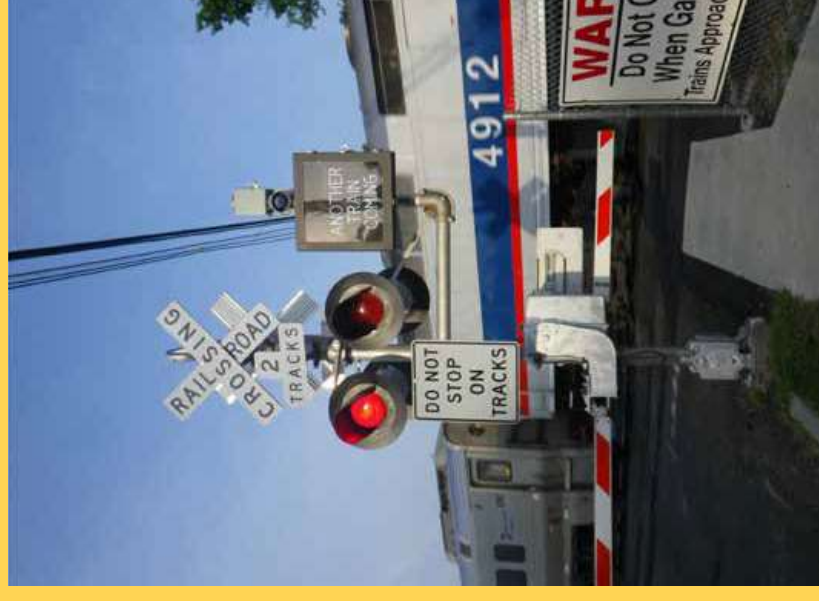
“Another Train Coming” system installed at Plauderville Station. Image: Marco DeSilva, Volpe Center
