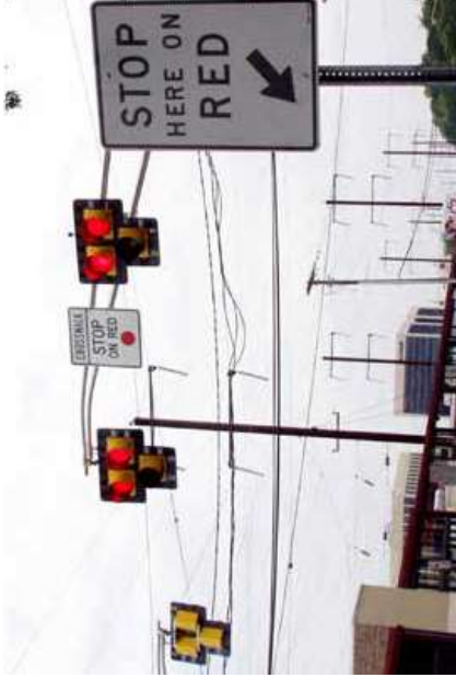
HAWK Signal across Route 27 to the Metropark Train Station. Image: NJDOT
