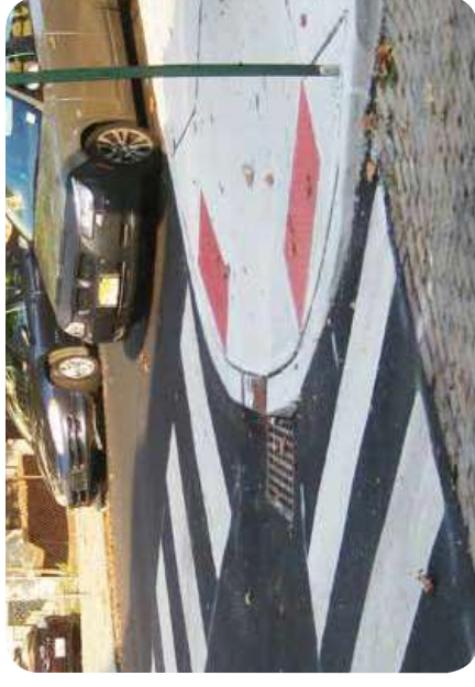
Intersections should have two perpendicular, ADA-compliant curb ramps per corner. Image: The RBA Group
