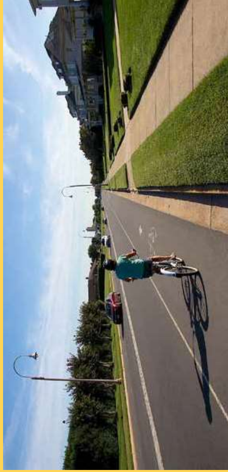
Ocean Avenue through Deal, NJ is an example of a Complete Street in a suburban setting with wide sidewalks and street lighting appropriate to the context. Image: Parsons Brinckerhoff
