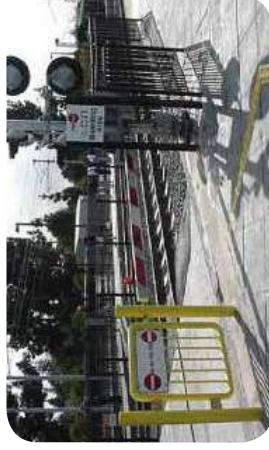
An emergency exit swing gate is used in conjunction with an automatic pedestrian gate. It is designated for use only as an escape route for a pedestrian that remains between the track and a lowered automatic pedestrian gate. Image: FHWA
