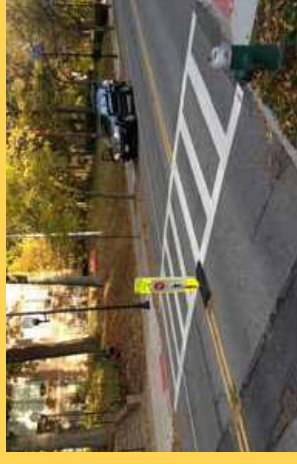
Newly painted high visibility, continental crosswalk and in-pavement “Stop for Pedestrian” crossing sign. Image: Arterial
