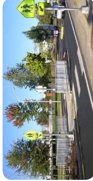
A median with a staggered crosswalk forces pedestrians to turn and face oncoming traffic before crossing the second half of the crosswalk. In order to curtail shortcutting and force pedestrians to follow the intended path, some medians may also have attractive fencing to corral pedestrians in the correct direction. Image: Oregon Department of Transportation
