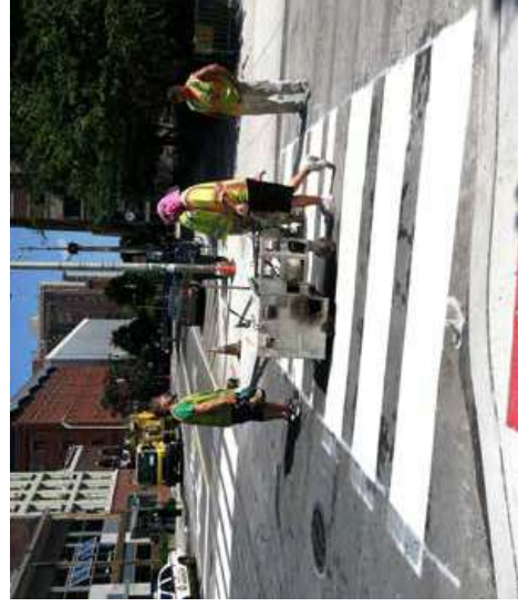
Installing high visibility crosswalks in Hoboken, NJ. Image: The RBA Group
