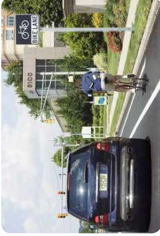
Narrowing the travel lanes on River Road in Hudson County, NJ allowed room for bike lanes. Image: NJ.com
