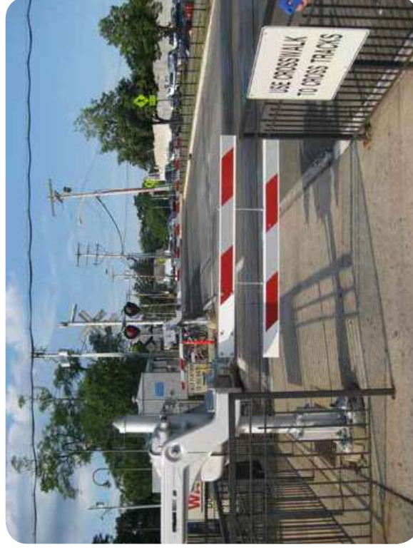
Pedestrian gate with “gate skirt” being tested at the Aberdeen-Matawan Train Station. Image: The RBA Group
