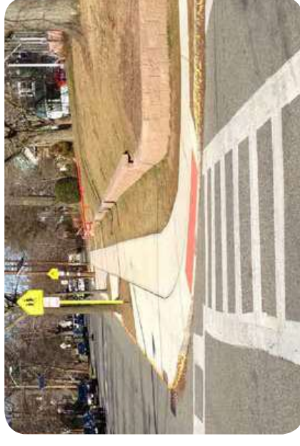
Diagonal curb ramps are not desirable because they force pedestrians into the intersection and are more difficult for visually-impaired people to determine the correct crossing location and travel direction. Image: Arterial
