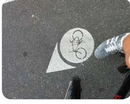
Bike Dots are pavement markings for signed bicycle routes. They are a tool to provide wayfinding. Image: TucsonVelo.com
