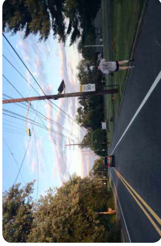
Burlington County has been striping 6-inch edge lines on shoulders along roadways with high bicyclist and pedestrian use, including this section of County Route 528 in a school zone in Bordentown Township. Image: NJDOT
