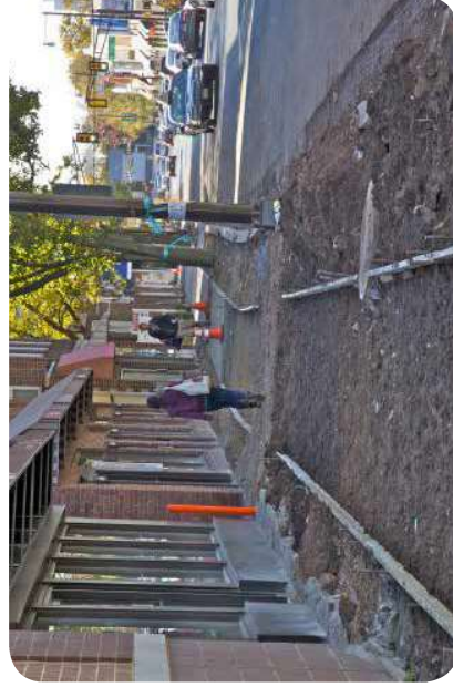
Sidewalk ready to be poured. Image: VTC
