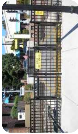
Example of a swing gate. Image: California Public Utilities Commission, Pedestrian-Rail Crossings In California
