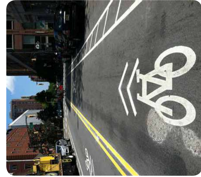
Newly-installed “sharrow” in Hoboken. Image: The RBA Group
