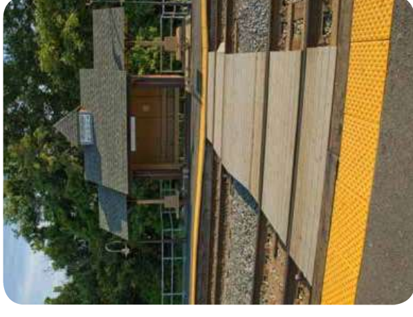
Example of visually contrasting surface materials at a pedestrian crossing. Image: FRA, Guidance on Pedestrian Safety at or Near Passenger Stations
