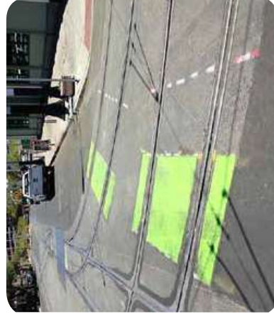
Green pavement markings in Tuscon, AZ indicate where cyclists may cross streetcar tracks at as close to perpendicular as possible. Image: bicycletuscon.com
