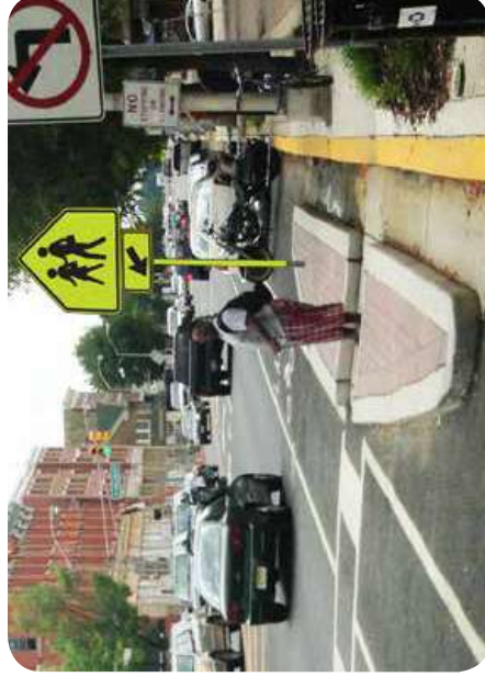
A mid-block storm-water curb extension example, Route 45 in Woodbury, NJ. Image: NJDOT
