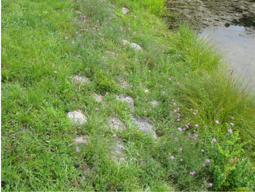
Photo No. 9: Closeup of the hand-placed riprap on the upstream slope.
