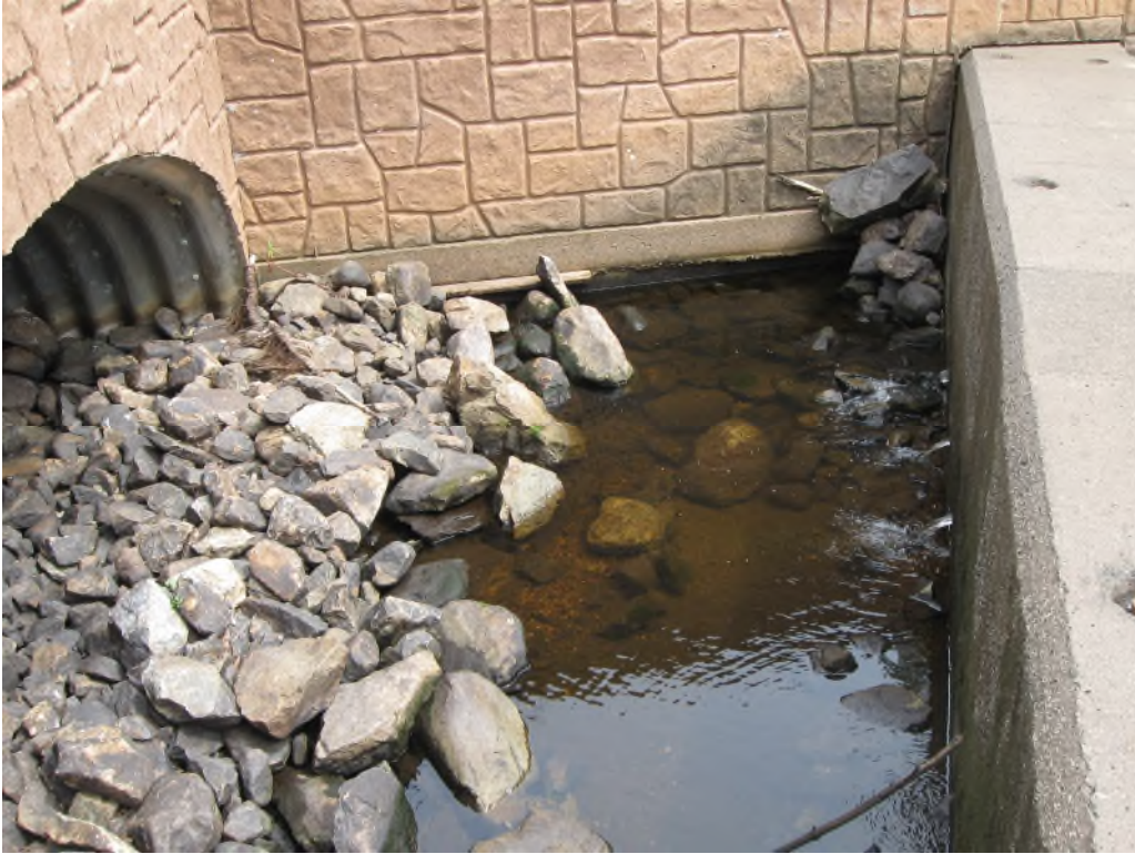
Photo No. 27: Transition area between the concrete step and the discharge culvert looking right. Note the scour hole in this area.
