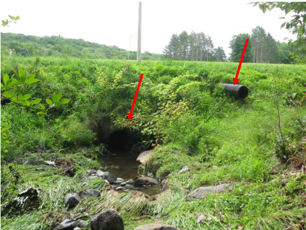
Photo No. 14: Left side lower downstream slope looking upstream at the storm drain discharge pipe and the low level outlet headwall. Note the overgrown conditions on the slope.
