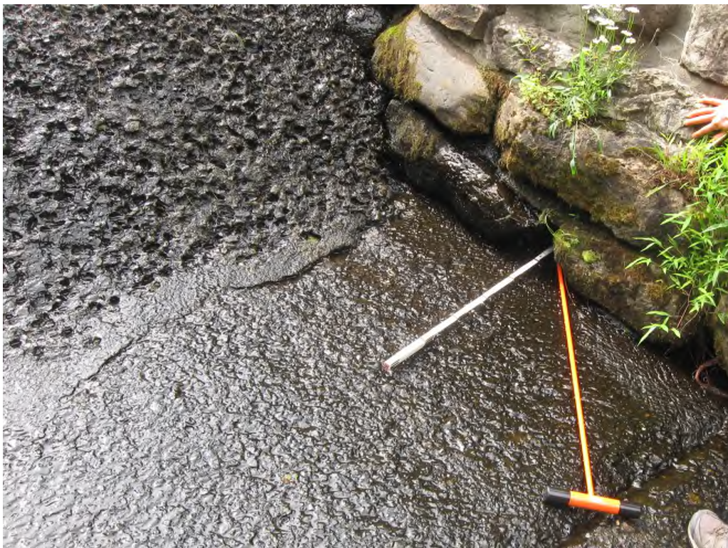
Photo No. 24: Closeup of the undermining along the base of the left side rock masonry spillway training wall.
