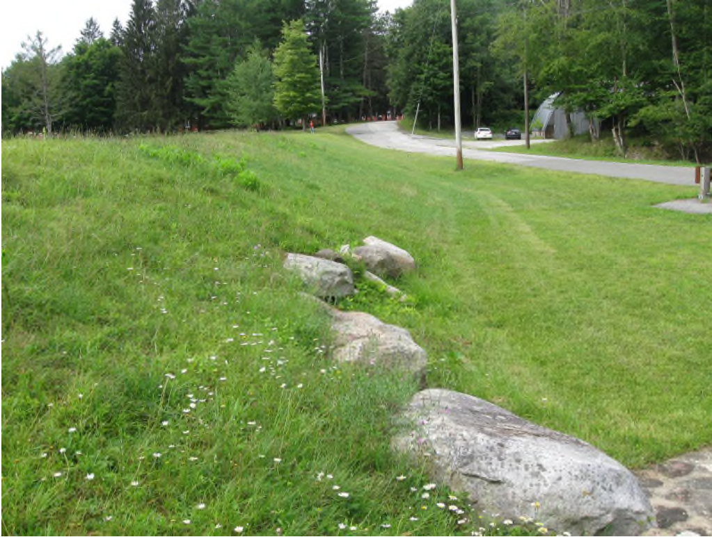
Photo No. 11: Left side upper downstream slope of the dam looking left. Note the large rocks along the bottom of the slope.
