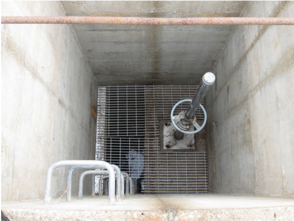
Photo No. 31: Interior of the low level outlet chamber located in the crest of the dam.
