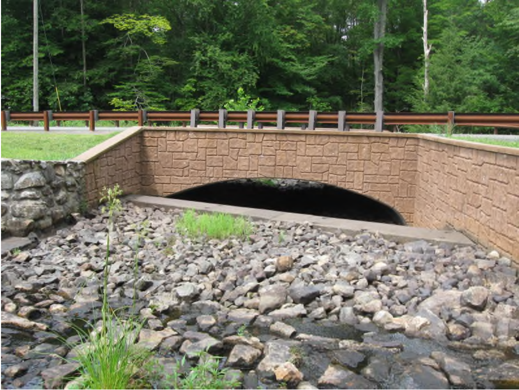
Photo No. 25: Looking downstream at the downstream riprap apron. Note the vegetation within the apron.
