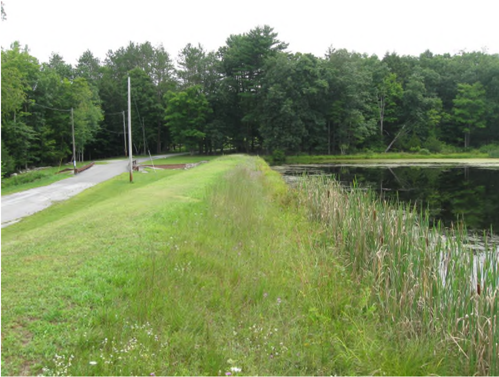
Photo No. 7: Left side upstream slope of the dam looking right. Note the tall vegetation on the slope.
