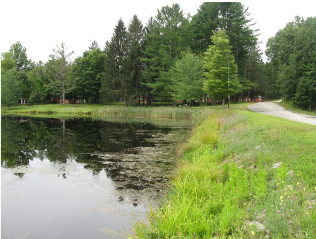
Photo No. 8: Left side upstream slope of the dam looking left. Note the tall vegetation on the slope.
