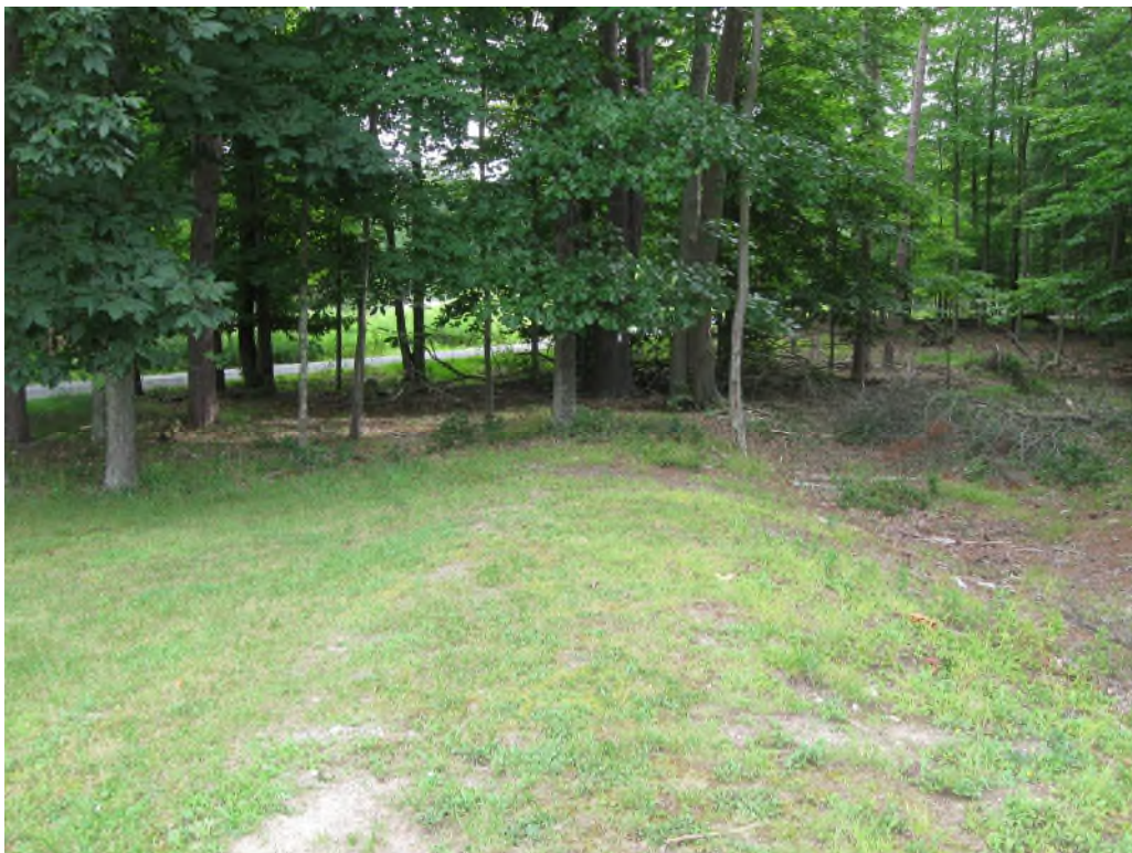
Photo No. 2: Right side crest of the dam looking toward the right abutment. Note the sparse grass cover on the crest.
