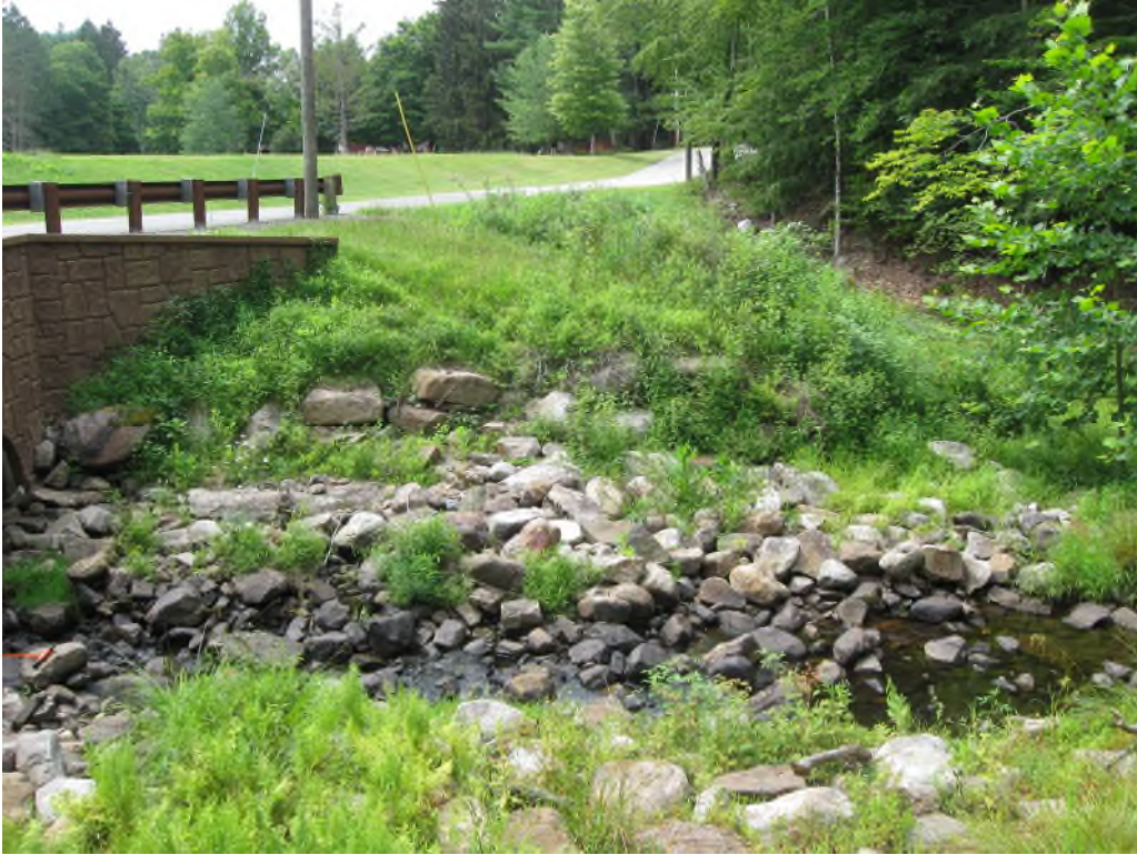
Photo No. 17: Left side lower downstream toe of the dam looking left. Note the overgrown conditions throughout the toe area.
