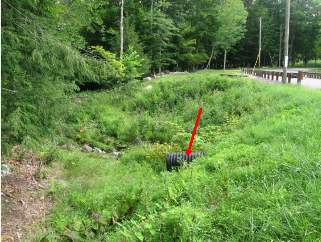
Photo No. 13: Left side lower downstream slope of the dam looking right. Note the overgrown conditions throughout the slope. Note the storm drain discharge pipe through the slope.
