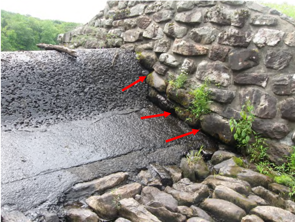
Photo No. 23: Left side rock masonry spillway training wall. Note that undermining has occurred along the base of the wall.
