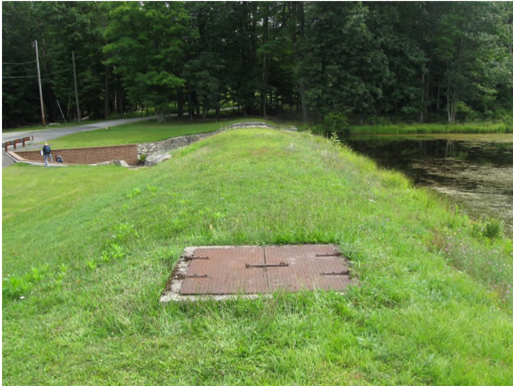
Photo No. 5: Closeup of the low level outlet chamber on the left side crest of the dam.
