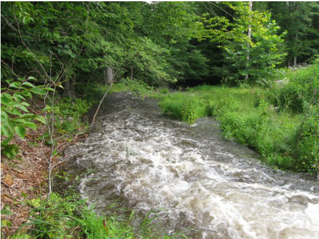
Photo No. 34: Low level outlet exit channel looking downstream during operation of the low level outlet. Note that the exit channel is narrow and shallow and does not have the capacity to pass the full flow from the low level outlet pipe.
