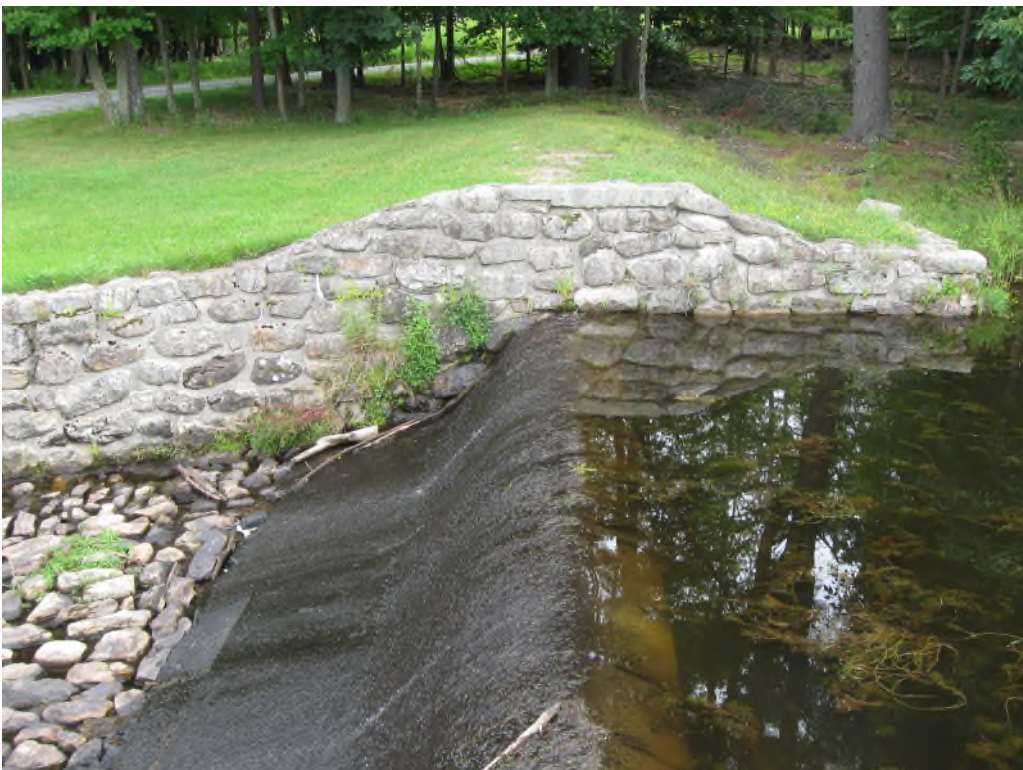
Photo No. 20: Spillway weir and entrance channel looking toward the right training wall.
