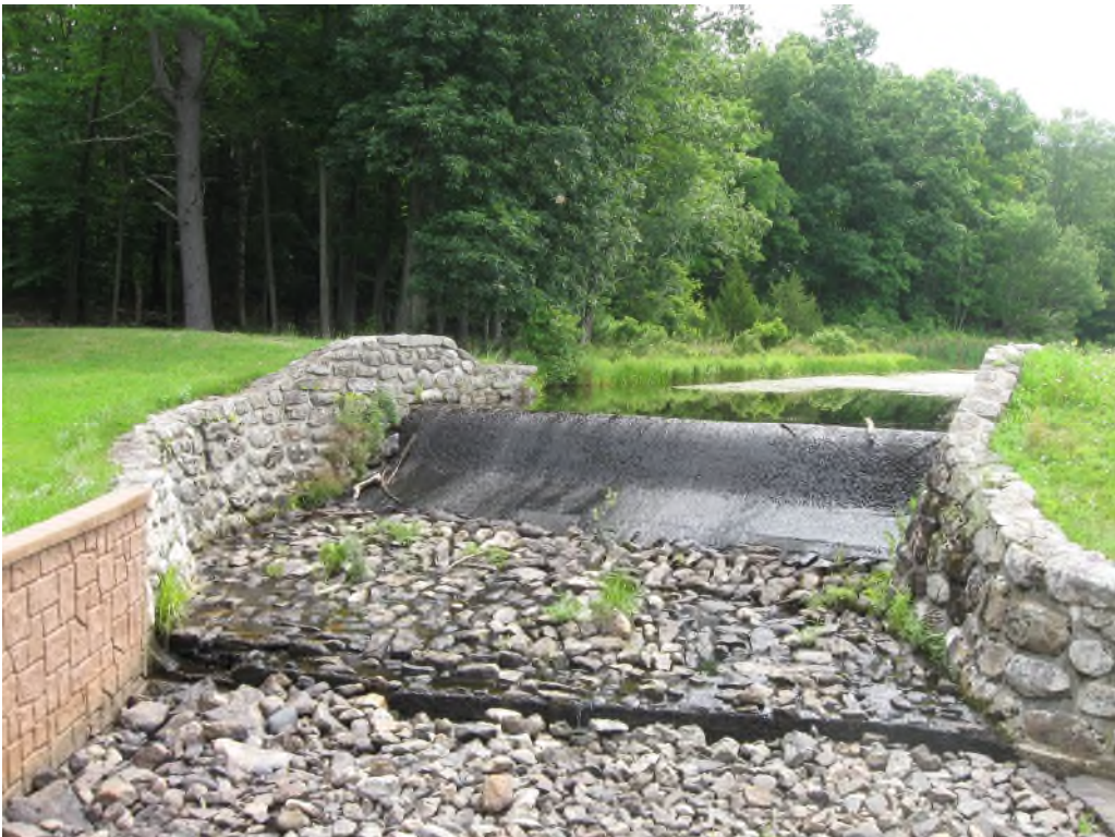
Photo No. 18: Spillway weir, rock masonry training walls and downstream riprap apron looking upstream.
