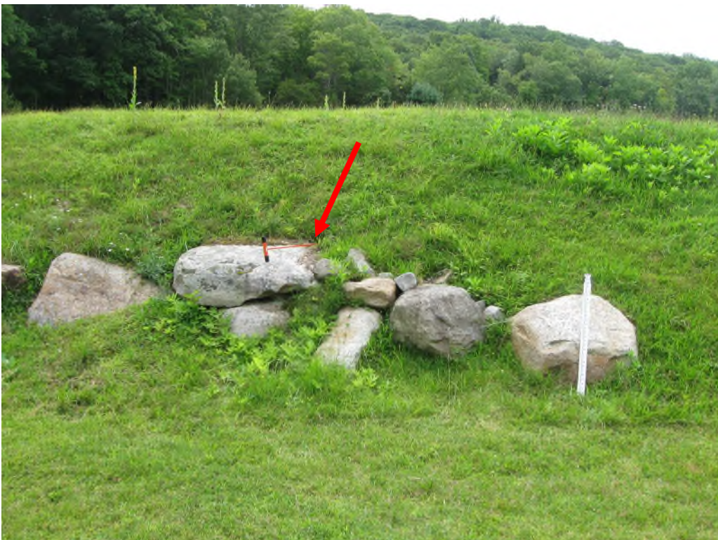
Photo No. 12: Closeup of large rocks along the left side upper downstream slope. Note the burrow hole above the rock.
