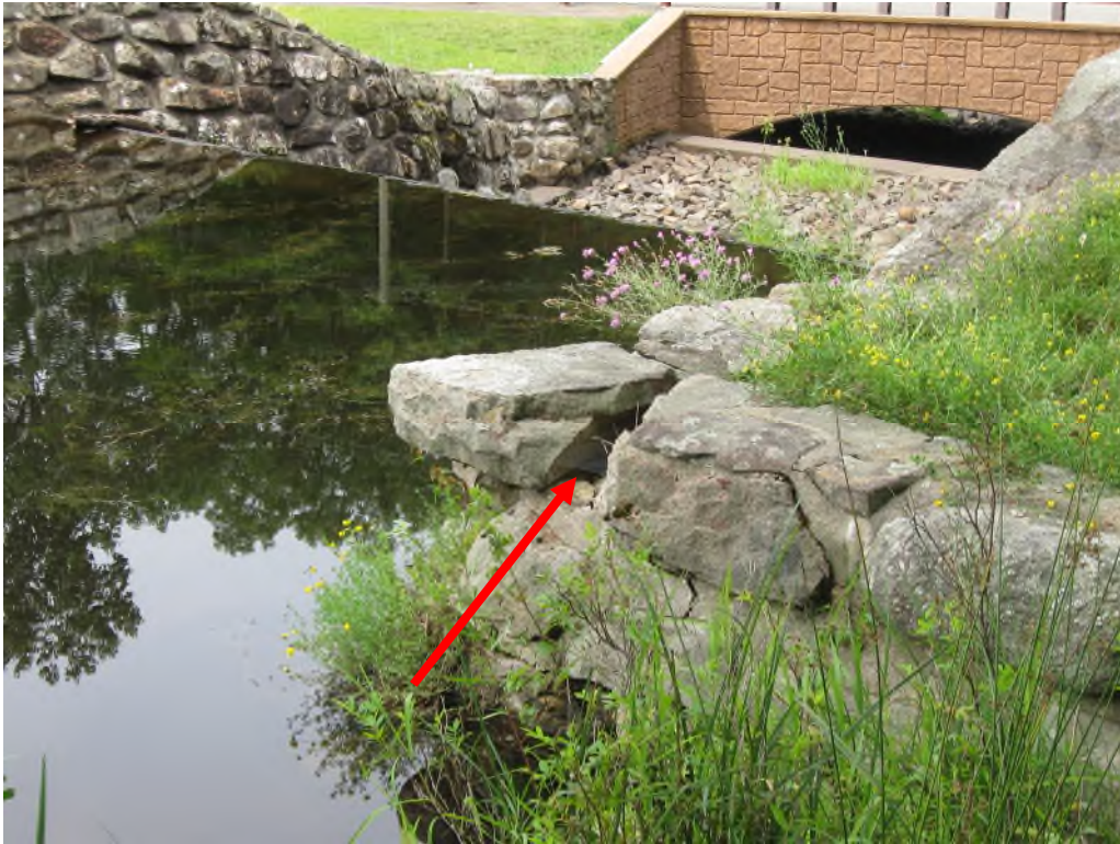
Photo No. 21: Closeup of the horizontal displacement of the upstream right rock masonry wall. Note that one of the stones was dislodged.
