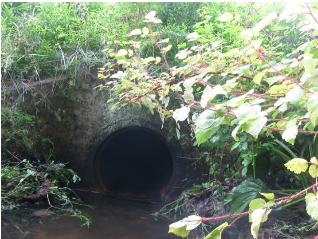
Photo No. 32: Closeup of the 24-inch diameter low level outlet discharge pipe and headwall. Note the thick vegetation surrounding the headwall and the standing water downstream of the pipe.
