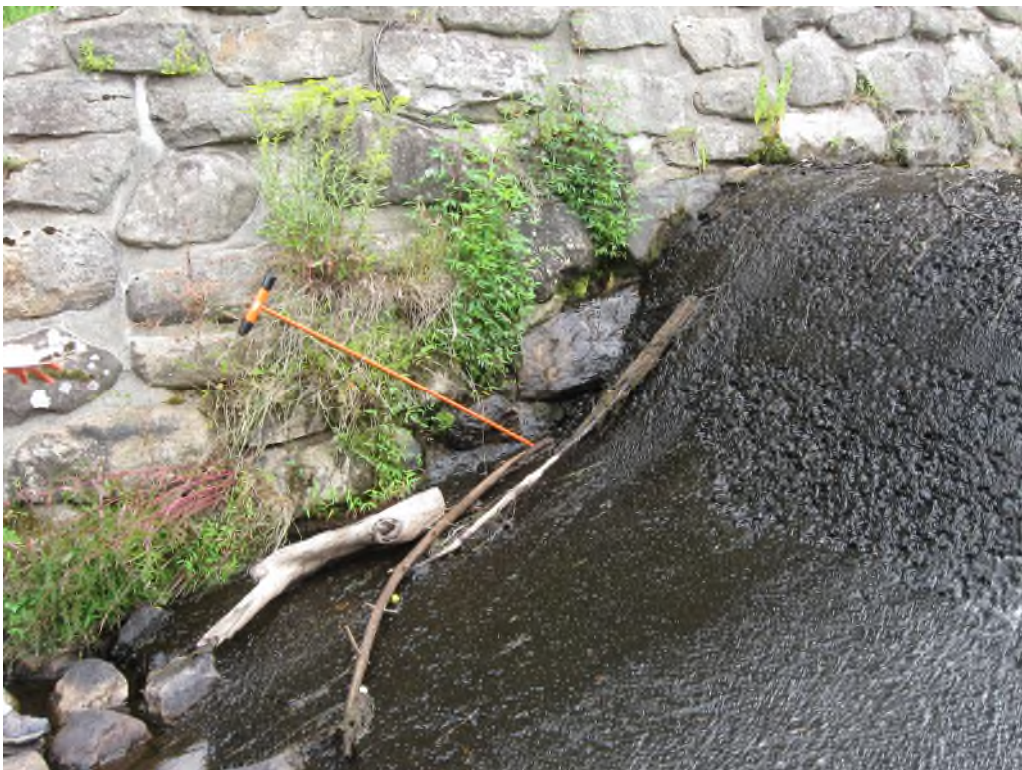
Photo No. 22: Right side rock masonry spillway training wall at the contact with the spillway. Note that minor leakage was observed through the wall at the contact with the spillway.
