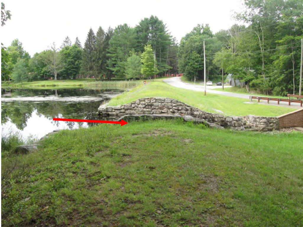
Photo No. 1: Right side crest of the dam looking left toward the spillway. Note the sparse grass cover on the crest and the low area adjacent to the right training wall.
