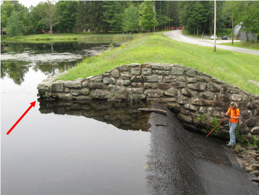
Photo No. 19: Spillway weir and entrance channel looking toward the left training wall. Note the missing stones in the upstream return of the left training wall.
