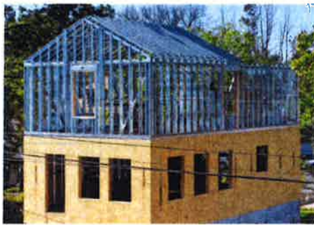
COURTESY BLUE DIAMOND CONTRACTING A new home in Keansburg may become the first in the state to qualify as a Fortified home, meaning the home is built to survive hurricanes and other high wind and heavy rain events.
