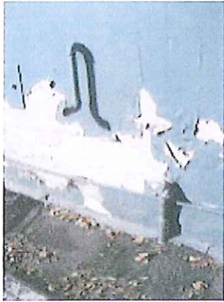
Former Natural Gas Connection (Meter Removed)
