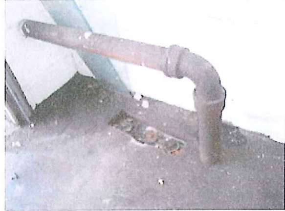
Sewer Vent and Clean-Outs
