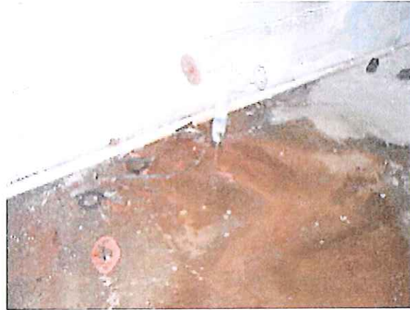
Water Service Pipe - Leaking
