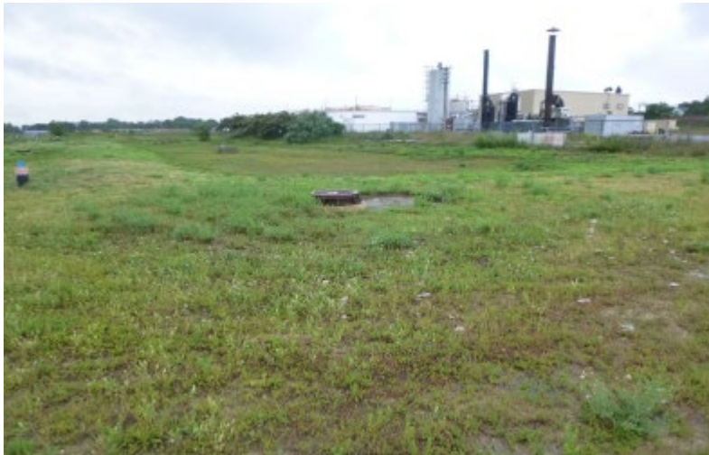
Photograph 5: View of a bioretention swale in the western portion of the Project Site. The BP groundwater treatment facility is visible in the background.
