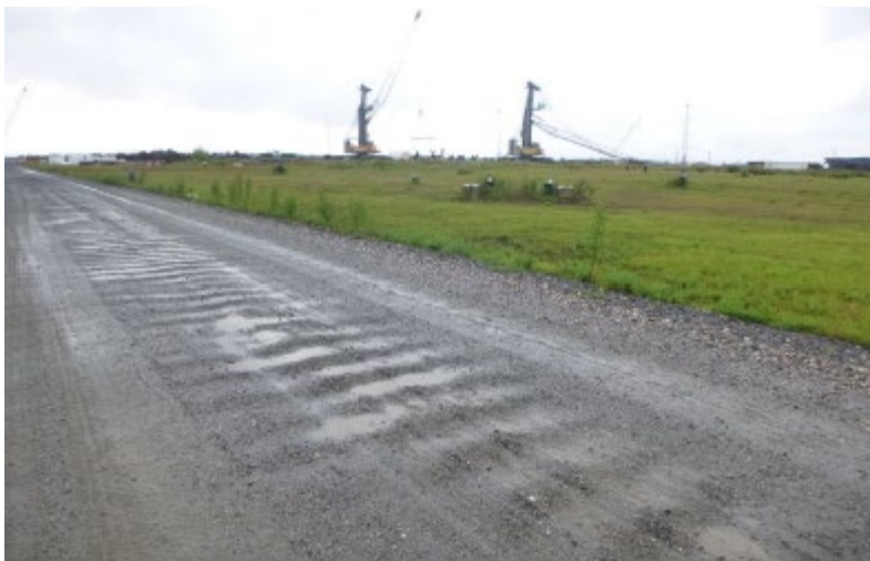
Photograph 8: Facing northwest, typical view in the northern portion of the Project Site. Two cranes atop the wharf are visible in the background.
