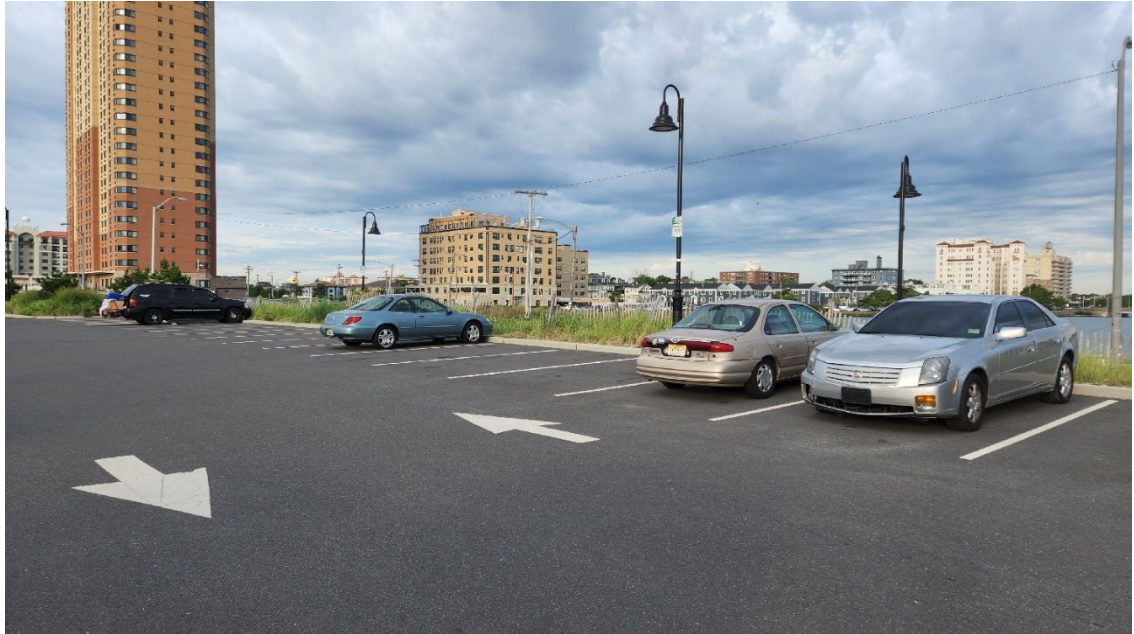
Photo 1.2-2 View of the Asbury Park Municipal Parking Lot Landfall in Vicinity of Proposed Boring
