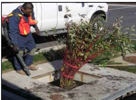
5. Clean area around Filterra
