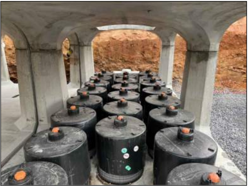
STORMPOD W/ CARTRIDGES (INSIDE VIEW)
