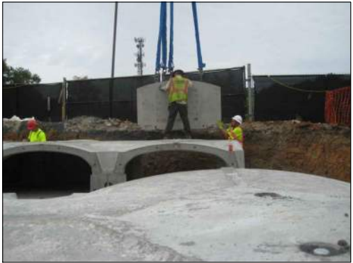
ENDWALL INSTALLATION
