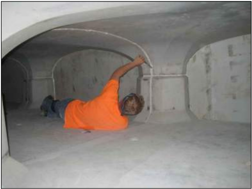
SEALING JOINTS
