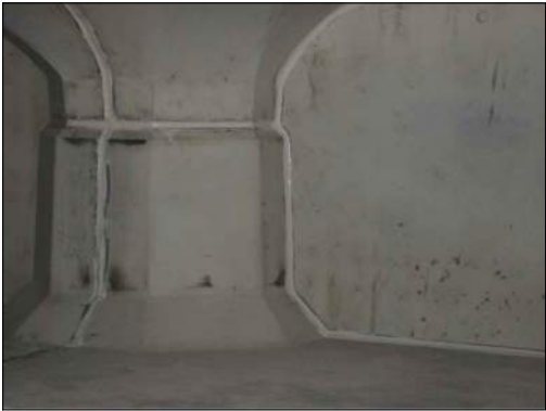
WATERTIGHT JOINTS (Tested to 17.25 psi hydrostatic pressure)
