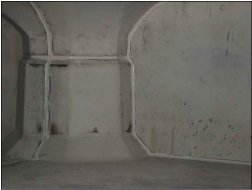
WATERTIGHT JOINTS (Tested to 17.25 psi hydrostatic pressure)
