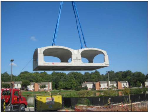
HANDLING (Base slab bolted to arch at factory)
