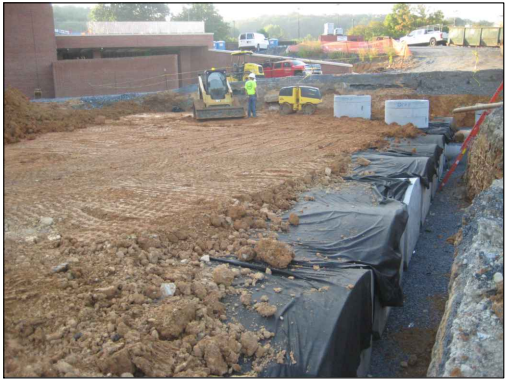
BACKFILL (On-site soils around perimeter & #57 stone in aquifers)
