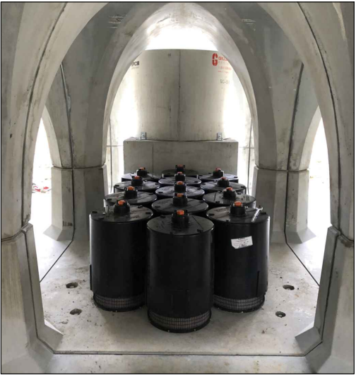
STORMPOD W/ CARTRIDGES (INSIDE VIEW)
