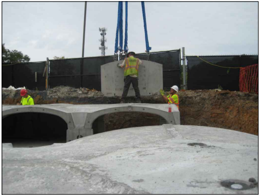
ENDWALL INSTALLATION
