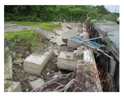
Photograph 5 – Example of former building foundation and general debris adjacent to North end of existing bulkhead.
