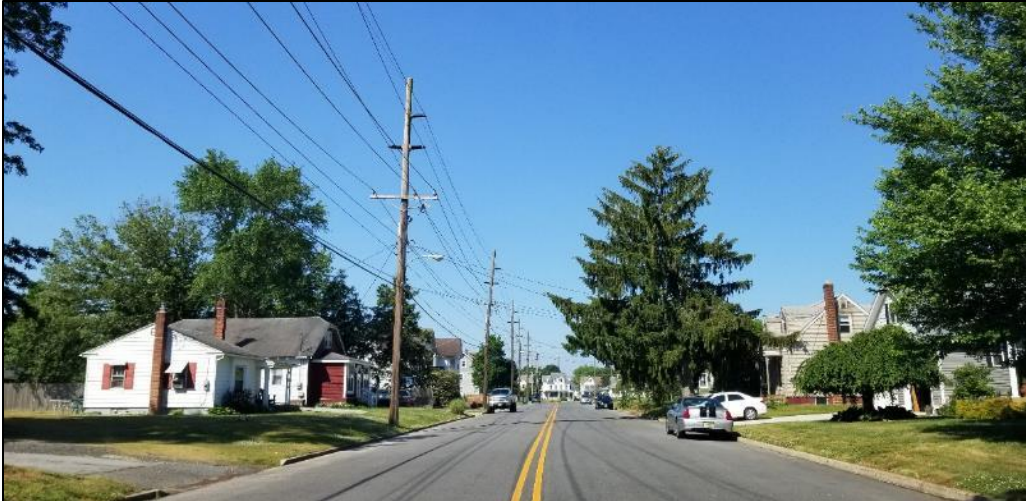
PHOTO 5: View west of ACE's inactive 69 kV transmission line along Lake Avenue in Quinton
