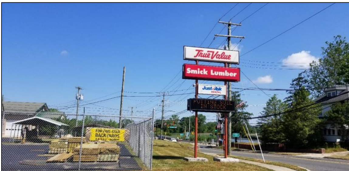
PHOTO 2: View north of the lumber yard located in Quinton with existing 69 kV line in the background
