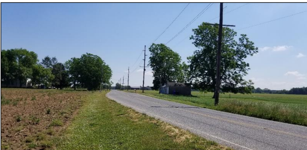
PHOTO 6: View east of the inactive Quinton-Hancock 69 kV transmission along CR 651
