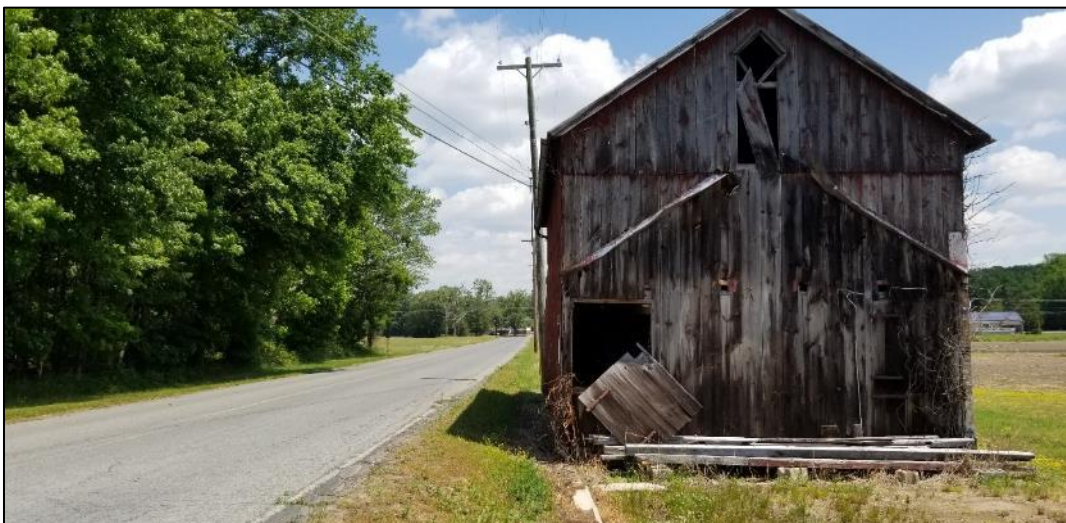
PHOTO 8: View east of a farm structure located close to the roadway edge with distribution lines overhead
