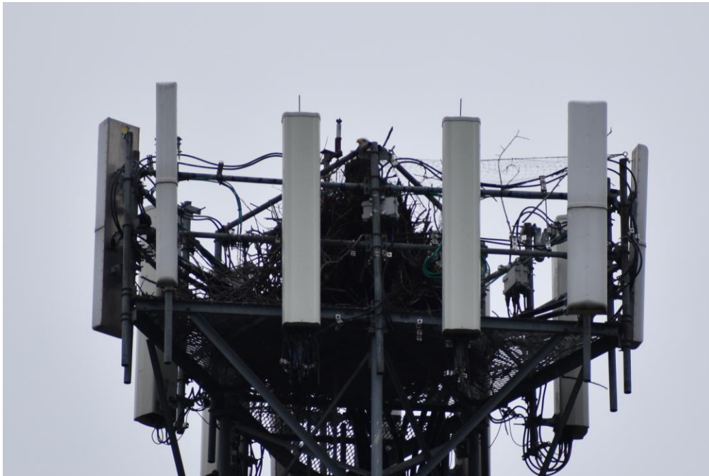
Photo 09: View of bald eagle nest "Alloway Creek C" located on communication tower NW of ROW
