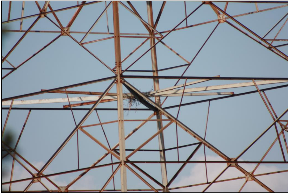
Photo 11: View of dilapidated osprey nest “Alloway Neck 2” below “Devil’s Gut” bald eagle nest within PSEG tower near Alloway Creek Neck Road
