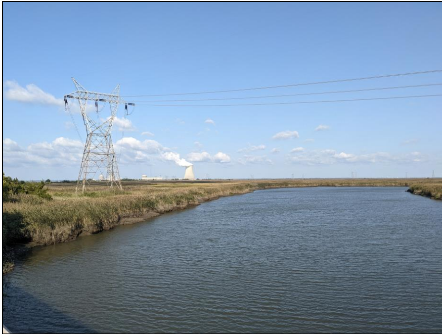
Photo 13: View of coastal conditions adjacent to Alloway Creek Neck Road
