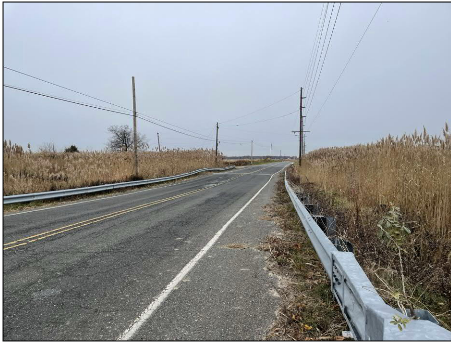
Photo 01: View of Phragmites estuarine marsh along project ROW
