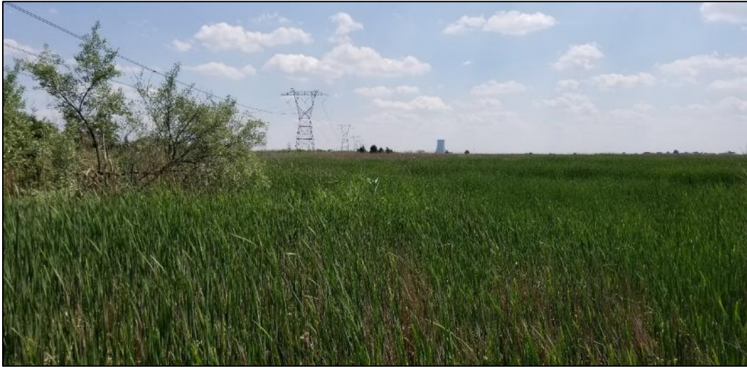
PHOTO 7: View south of the Hope Creek-Keeney 500 kV transmission line and surrounding tidal marsh
