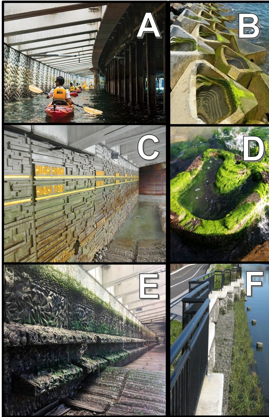
Figure 5. The case studies analyzed for this study showcase the six Design Elements. (A) Allowing Light Penetration is accomplished through translucent panels incorporated into the cantilevered walkway at Seattle Seawall ( credit: City of Seattle ). (B) Using Alternative Materials is realized through the use of
