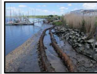
BEFORE: Day of installation of coconut-fiber (coir) logs and mats in New Jersey's Heislerville Fish and Wildlife Management Area in May of 2010.
