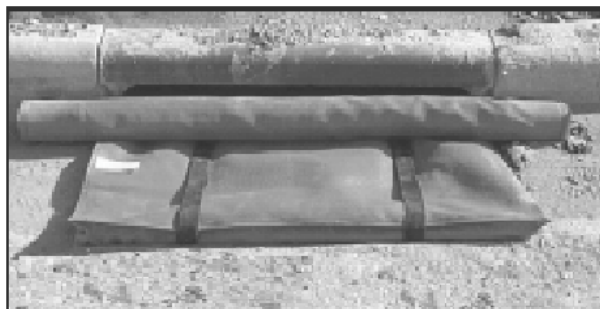
Storm drain inlets blocked during bulk fuel transfer.
