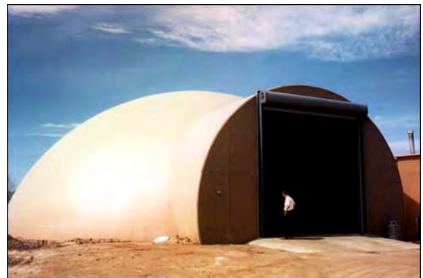
Monolithic, or shotcrete dome.
