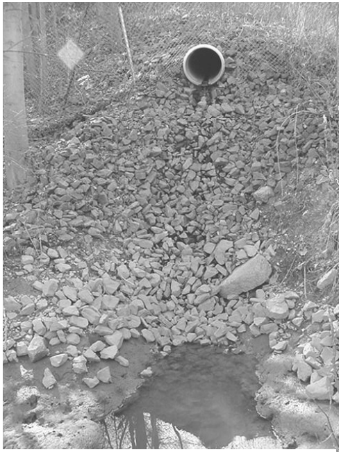
Scour holes are caused by excessive velocity of the discharge. Riprap may help dissipate the flow, reducing damage to the stream bank.
