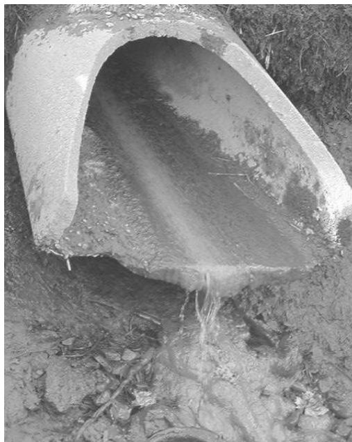
Physical observations of the discharge for turbidity, staining, odor, and color can help determine the source of the illicit connection.
