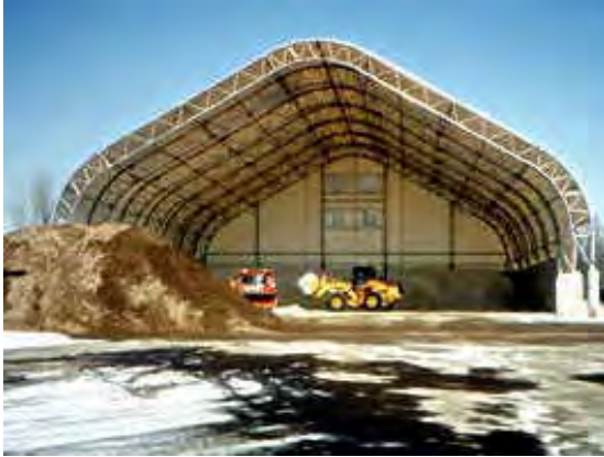
This three sided storage structure does not comply with the permit minimum standard.
