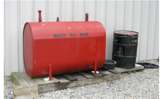
This AST should be on an impervious pad and within secondary containment.
