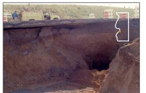
Figure 6. Another view of the sinkhole from Figure 5 that opened during construction of I-78 in the Phillipsburg area in 1989. The area above this sinkhole collapsed just before the highway was due to open and delayed the highway opening by several months. Diagonal lines illustrate the report of human activity on sinkhole development. Photograph by H. Kasabach. Star shows location of photograph in map area.
