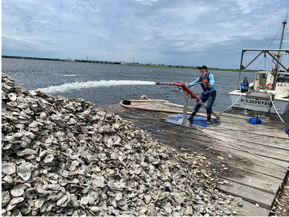
Figure 21. Shell being planted over the Mullica River oyster reefs by MRA staff using the new water cannon
