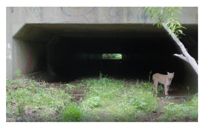
Oversized stream culverts that include dry ground are important safe passageways for terrestrial wildlife, and they're encouraged in the new Infrastructure Act. Here, a Bobcat crosses below a busy six-lane highway in north Jersey. In time, we'd like more culverts to double as animal underpasses. *Trail cam photo by our volunteer, Melissa McCutcheon*
