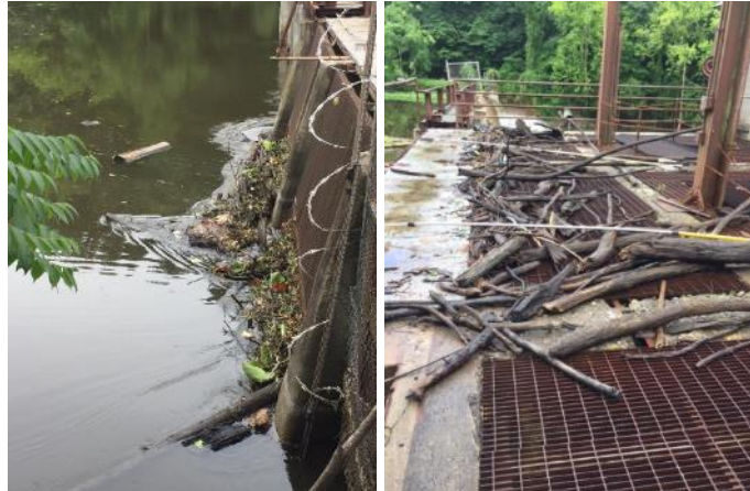
Clogged trash racks of decommissioned hydro-electric facility at Columbia Lake.
