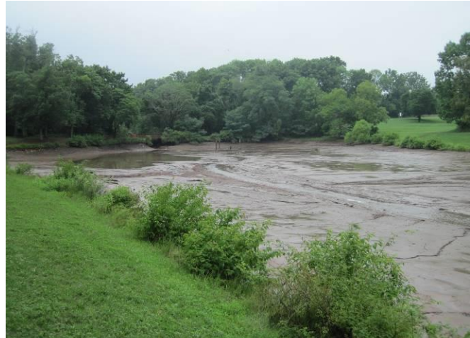
Deer Path Park Pond reduced from 2 acres to a stream channel and a small shallow pool after its dam failed in 2016
