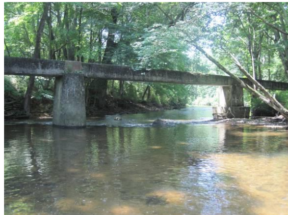
Claremont Stretch fiber optic crossing.
