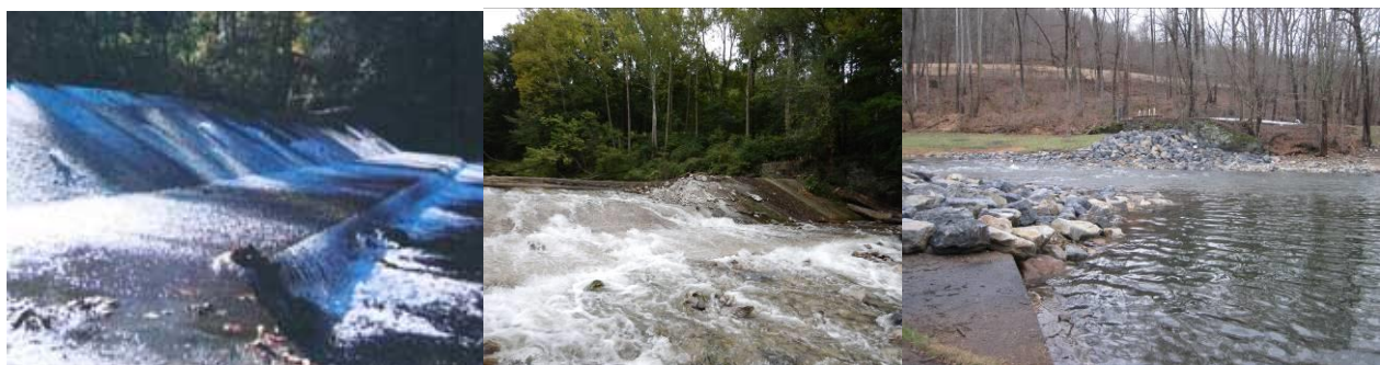
The three photographs above represent various stages of removal of the Hughesville Dam. (left: pre-removal, middle: after initial breach, right: complete dam removal)
