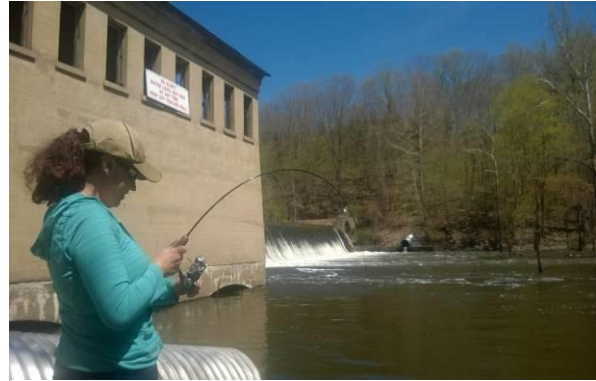
Columbia Lake Dam
