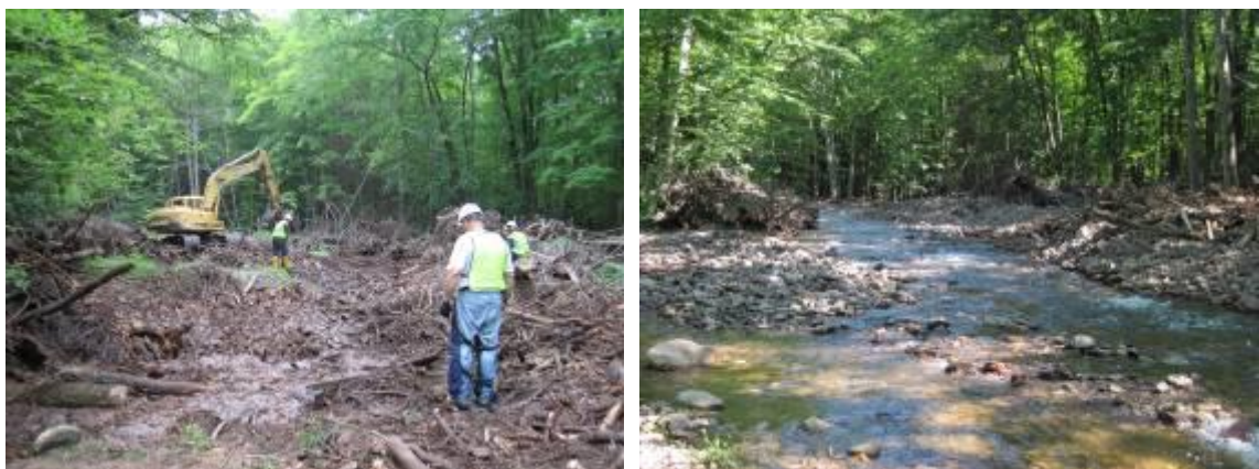
Impeded flow of the Big Flatbrook during woody debris removal (left) and restored flow via the main channel following debris removal after (right).
