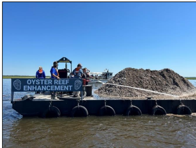
Staff use barge and water cannons to plant recycled shells onto New Jersey oyster reefs.
