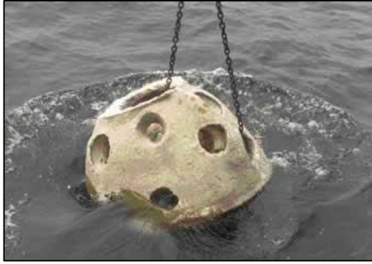
A reef ball is deployed on the Cape May Artificial Reef.
