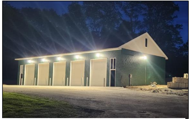
The impressive new 5-bay garage at Hackettstown.
