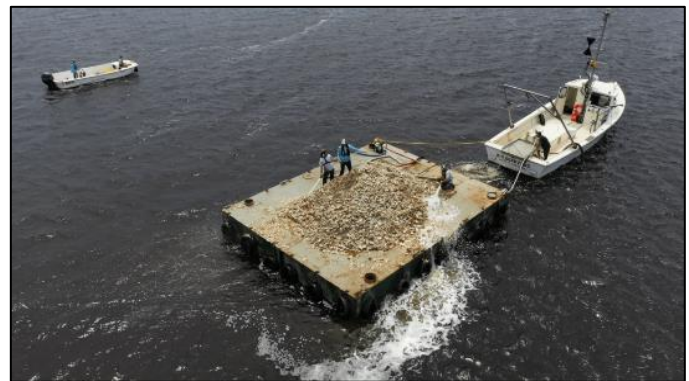
A barge and water cannons are used to plant recycled shells onto New Jersey's oyster reefs.
