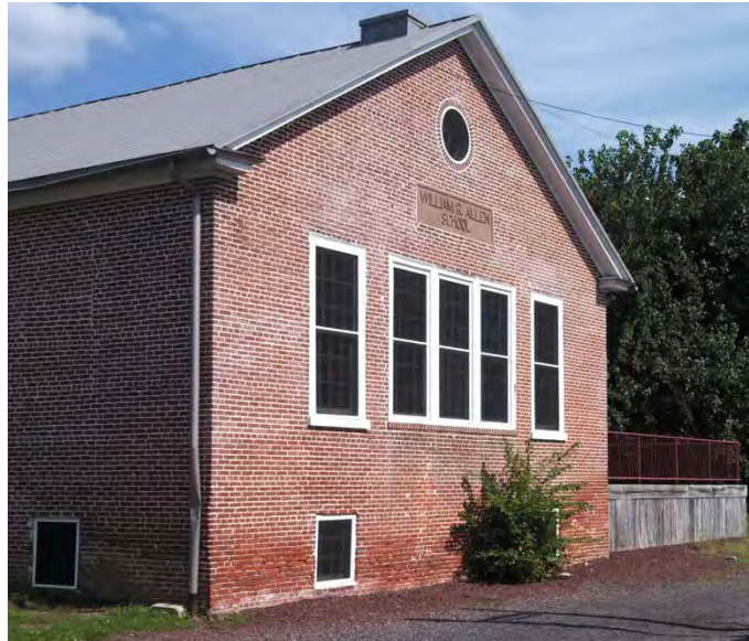
Figure 82: West Elevation of the William R. Allen School. This is part of the original building, c. 1910.
