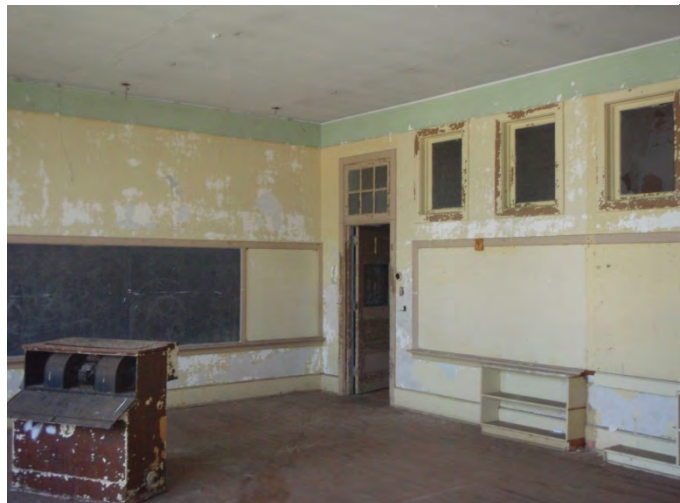
Figure 92: Classroom in relatively good condition.
