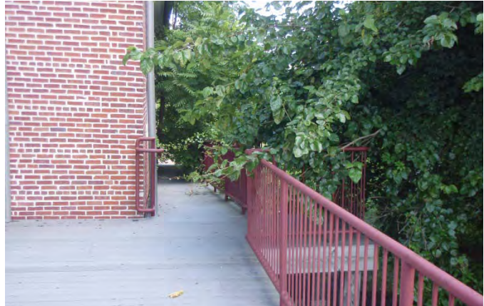
Figure 97: The HC access ramp constructed at the rear of the William R. Allen School.
