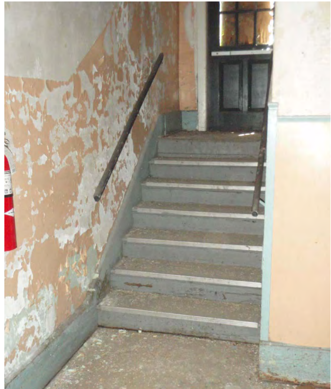
Figure 98: Existing egress stairs that connect the basement and first floors to the exterior.
