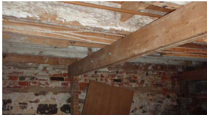
Figure 42: Image of structural reinforcing and "sistering" of damaged floor joists in the basement of the Hoskins House.
