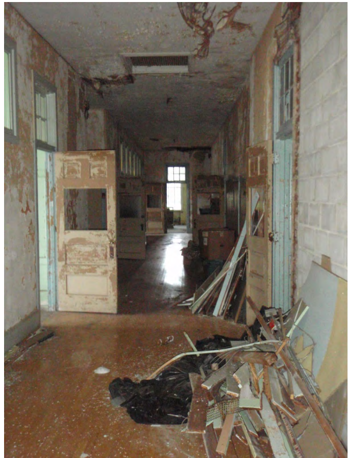
Figure 95: Main corridor of the first floor of the William R. Allen School.
