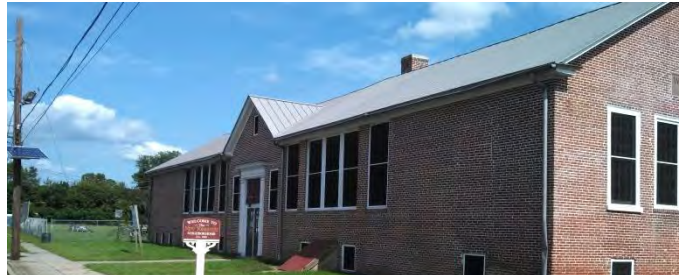
Figure 83: Front of the William R. Allen School on Mitchell Avenue in Burlington, NJ. The original building is to the right.
