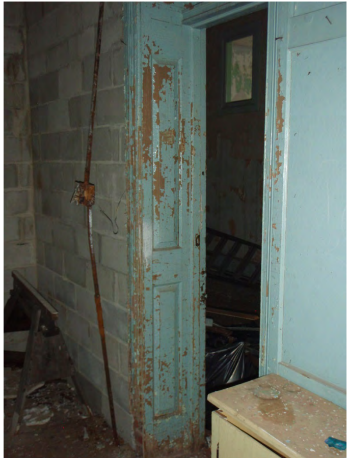
Figure 99: Trim and molding details in the William R. Allen School.
