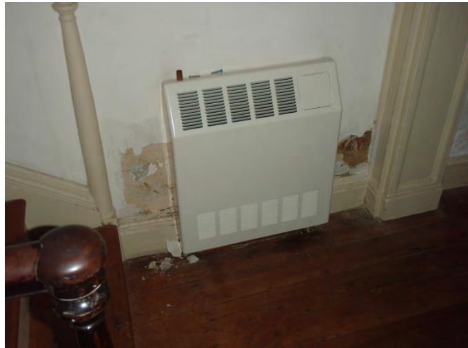
Figure 37: Relatively severe plaster damage in the entry hall, first floor of the Hoskins House.
