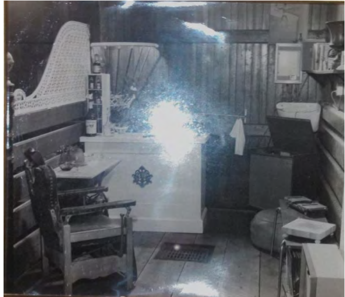
Figure 62: Carriage House interior prior to restoration, when it was used as an antique shop. The original stable separation walls are apparent. Photo is located in the Carriage House.
