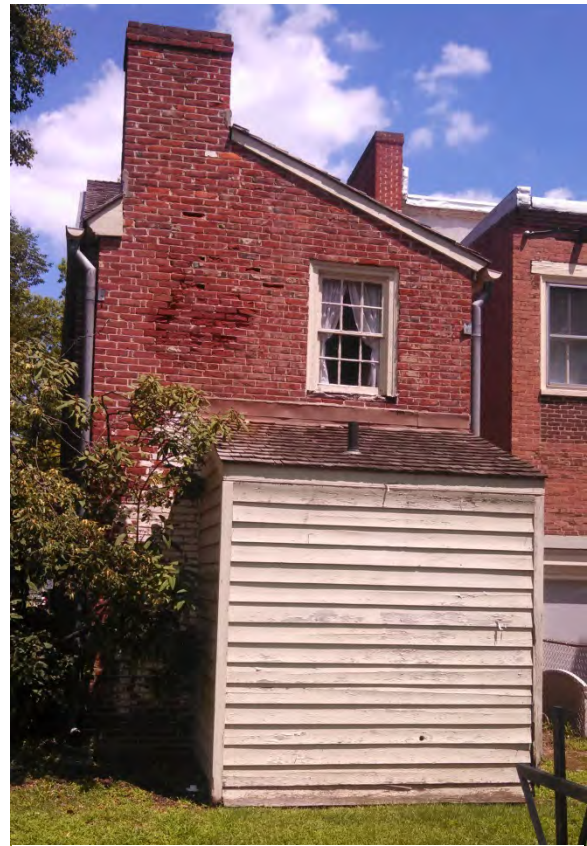
Figure 25: Rear of the Hoskins House.
