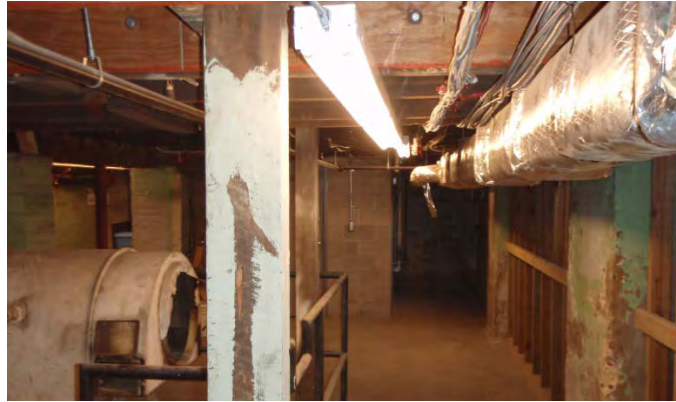
Figure 59: Image of structural reinforcing in the basement of Lyceum Hall.
