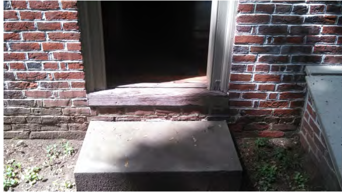
Figure 21: All of the doors at the Quaker Schoolhouse have blue-stone stoops, preventing HC access.
