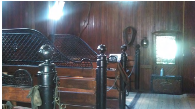
Figure 77: Beaded board paneling on the first floor in good condition.
