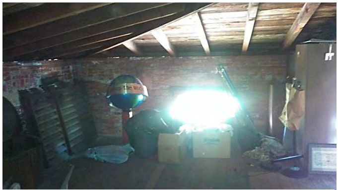
Figure 78: Exposed rafters above the stable area.
