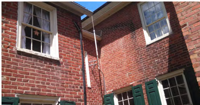
Figure 29: Image of rear windows and trim in relatively good condition.
