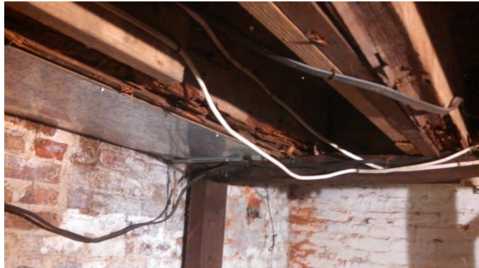
Figure 79: Sistering and structural reinforcement in the basement of the Carriage House.
