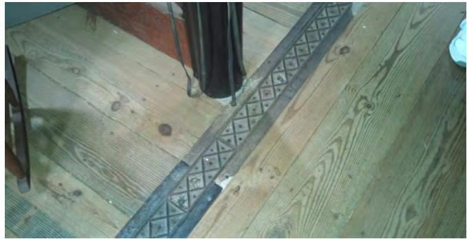
Figure 74: New flooring in the stable area.
