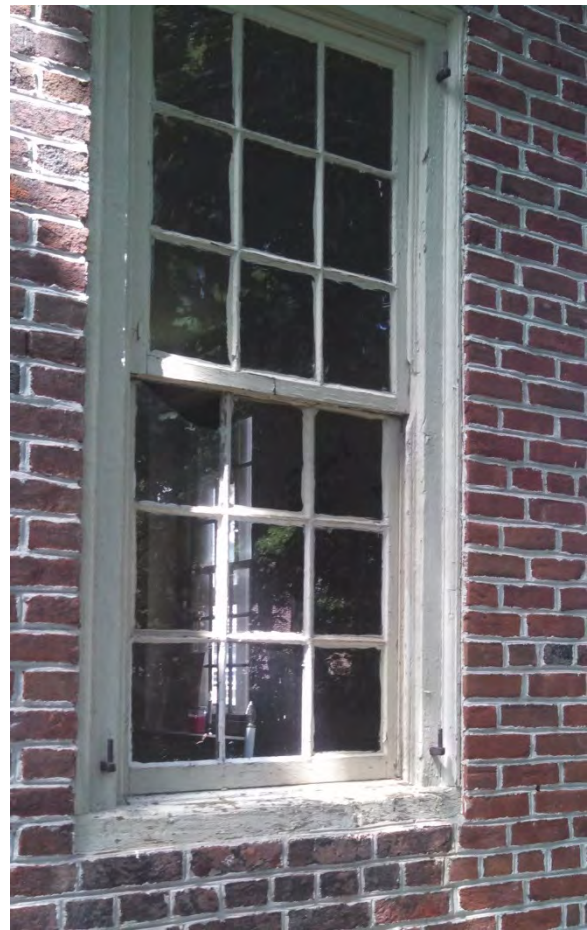
Figure 10: Typical condition of exterior window at the Quaker Schoolhouse.
