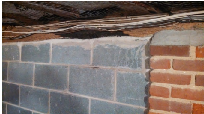
Figure 20: New bearing wall in basement of Quaker Schoolhouse, showing sill plate that has been reinforced.
