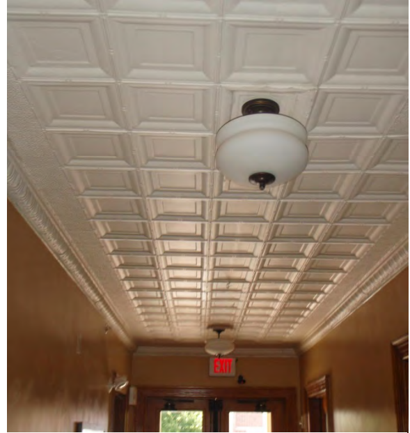
Figure 48: Pressed tin ceiling in first floor corridor of Lyceum Hall.
