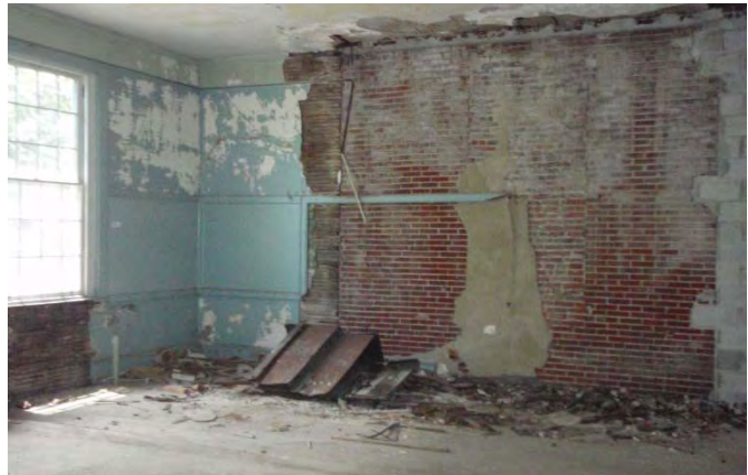
Figure 96: Repaired bearing wall at the William R. Allen School.
