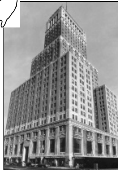
NATIONAL NEWARK & ESSEX BANKING COMPANY BUILDING
