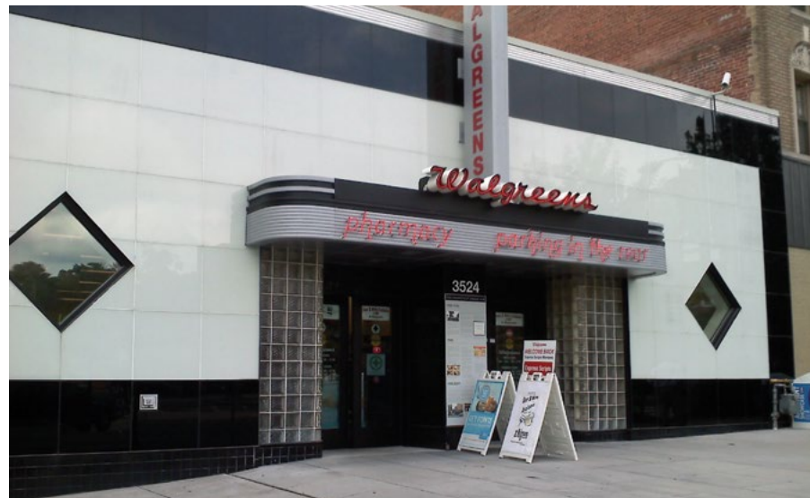
[11] (a) Some of the materials on the front of this historic building had been previously replaced, but the façade retained its essential distinctive features and design. (b) A vintage postcard of the building (far left) provided sufficient documentation to restore the façade to its historic 1945 appearance, using spandrel glass as a replacement for the original Carrara glass (c). Photo (b): Courtesy Kelsey & Associates.
