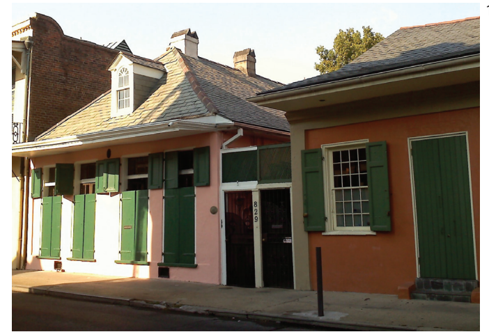
[10] Wood shutters provide natural light when open and keep interiors cool when closed in historic residential buildings.
