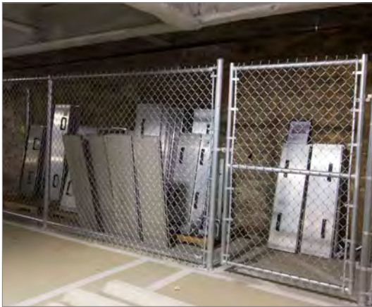
Window and door barriers and shields for dry floodproofing are generally inserted into pre-installed channels flanking window and door openings. They must be individually labelled and stored onsite in a convenient location, and installed by trained personnel immediately preceding a flood event.
