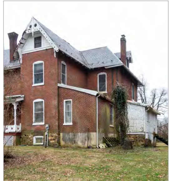
A poorly maintained building is less likely to withstand flood damage than a well maintained building. If the structural system is compromised, it will be more difficult and more costly to elevate or relocate.
