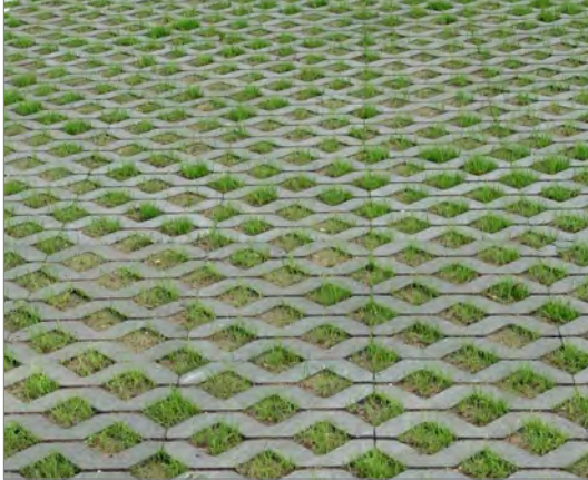
Pervious paving reduces stormwater runoff by encouraging absorption into the soil.
