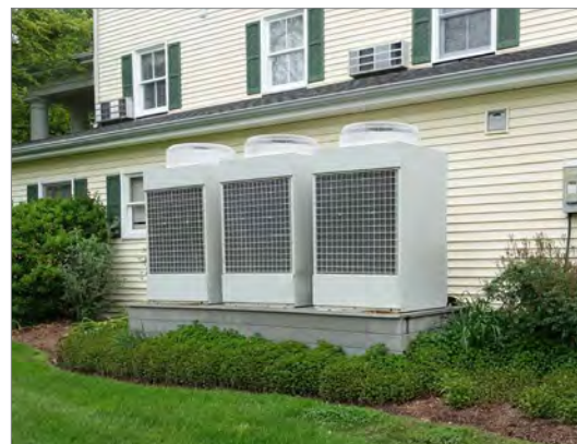
Elevating building systems and equipment can reduce damage from rising water and expedite repairs following a flood event. Appropriate screening is recommended.
