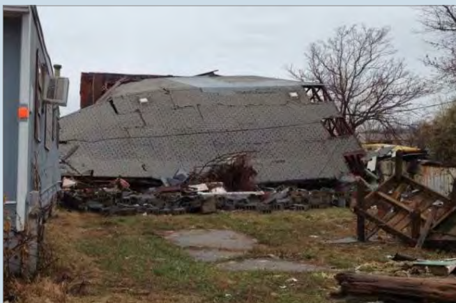
Criteria 2: The roof has collapsed on this Highlands, Monmouth County building. It is also likely that it meets Criteria B for pancaking. (Photography courtesy of the NJ HPO.)
