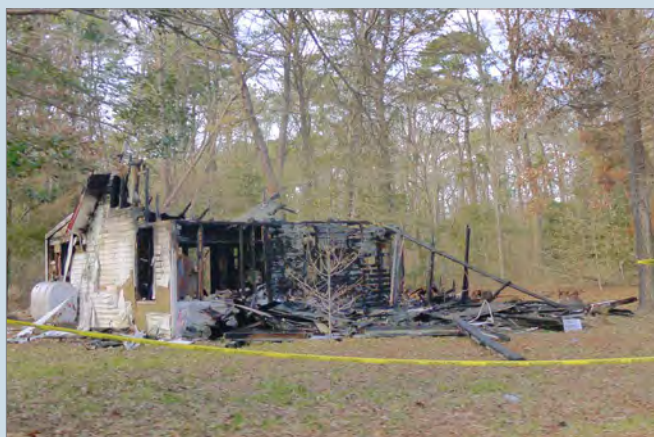
Criteria C: Fire damage has structurally compromised this building in Brick, Ocean County. (Photography courtesy of the NJ HPO.)
