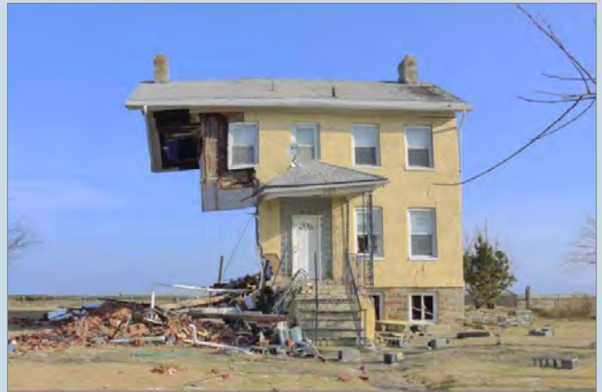
Criteria 3: This Union Beach, Monmouth County residence is missing one or more of its complete elevations. (Photography courtesy of the NJ HPO.)
