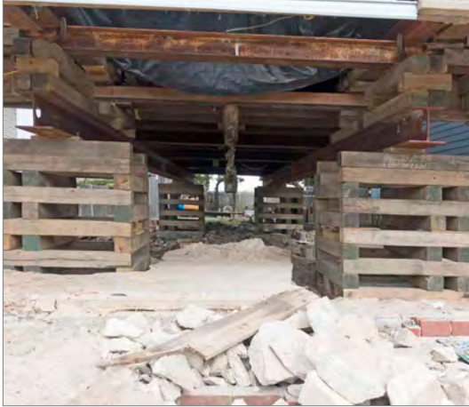
All systems must be disconnected prior to lifting the building off of its foundation.
