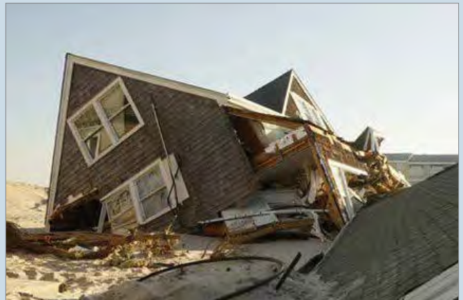
Criteria 4: More than 50% of this residence in Mantoloking, Ocean County is off of its foundation. (Photography courtesy of the NJ HPO.)
