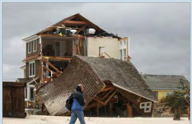
Criteria 5: This residence in Mantoloking, Ocean County is split or sheared. (Photography courtesy of the NJ HPO.)
