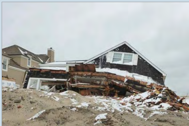
Criteria B: This residence in Mantoloking has pancaked, with the lower floors resting on the ground below. (Photography courtesy of the NJ HPO.)
