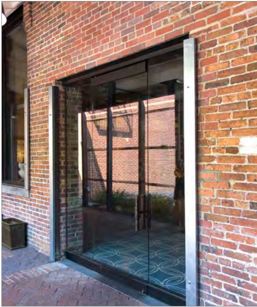
Window and door barriers and shields for dry floodproofing are generally inserted into pre-installed channels flanking window and door openings. They must be individually labelled and stored onsite in a convenient location, and installed by trained personnel immediately preceding a flood event.
