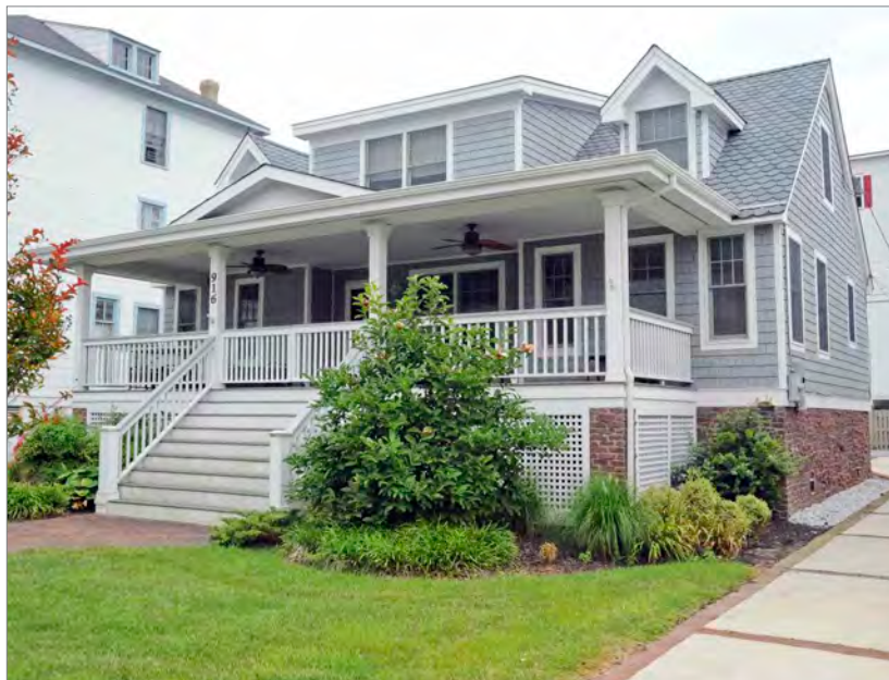
Square lattice provides foundation screening between the piers. The use of diagonal or square lattice should be appropriate for the building's style. The central stair maintains the orientation to the front door and the brick foundation of the house includes flood vents at the side elevation facing the driveway.
