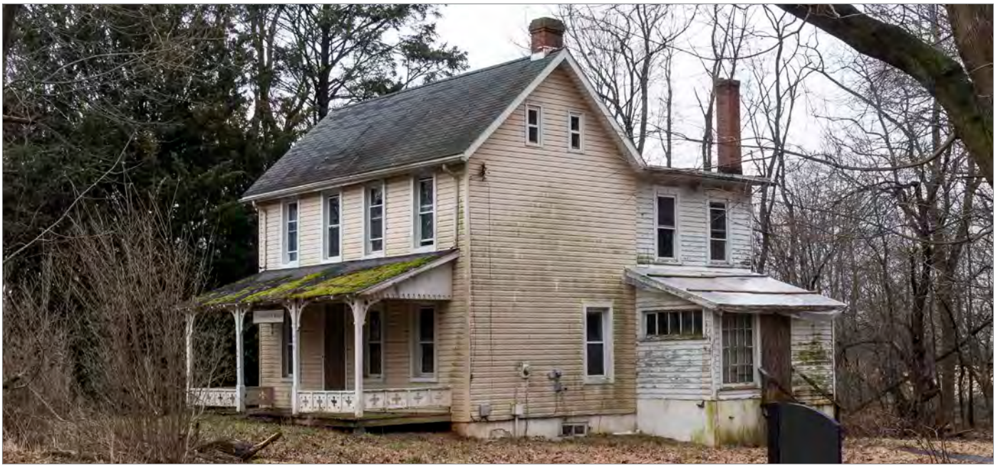
Poorly maintained buildings are more susceptible to damage from flooding and may require stabilization prior to elevation.
