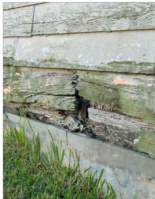
Wood, particularly unpainted wood near the ground, is highly susceptible to damage when exposed to flood water.
