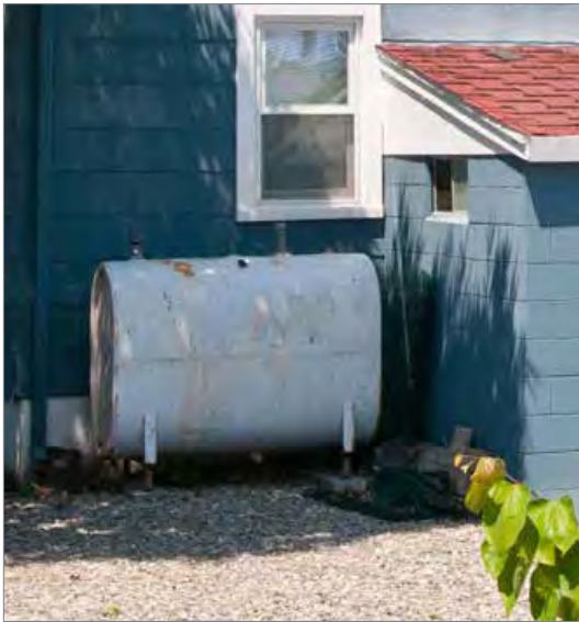
Propane tanks can provide an alternative fuel source however, they should be secured to prevent floatation in a flood event.
