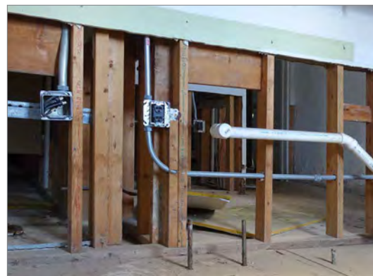
Interior drywall was removed and electrical outlets and plumbing connections were raised following a flood.
