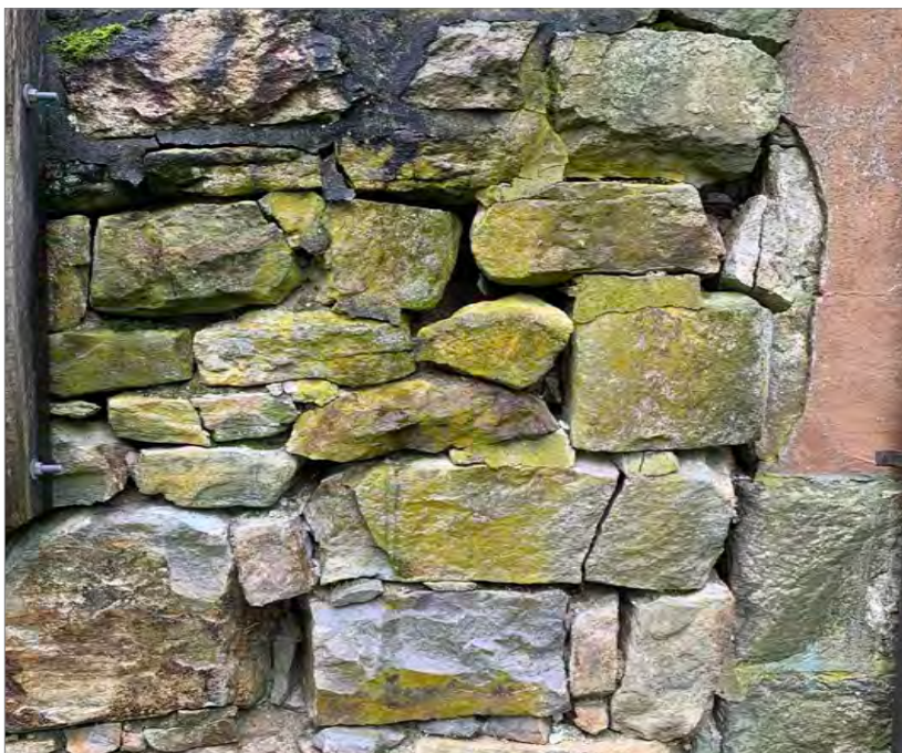
Proper maintenance can impact the flood resilience of materials. Although the stone may be an acceptable flood resistant material, the lack of mortar provides a path for flood water ingress.
