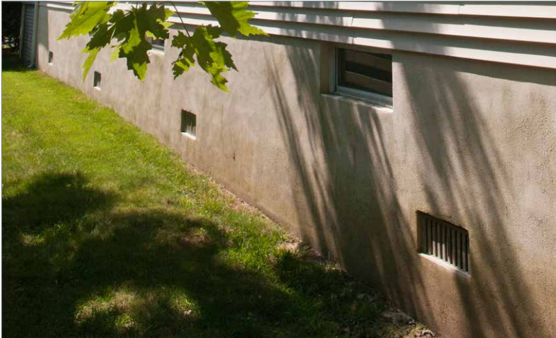
Flood vents, such as those located along the foundation, allow the free passage of water in and out of a closed foundation or building.
