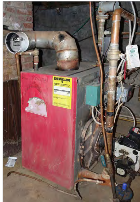
Building systems and equipment are often located in basements where they are highly susceptible to flood damage, necessitating costly replacement.
