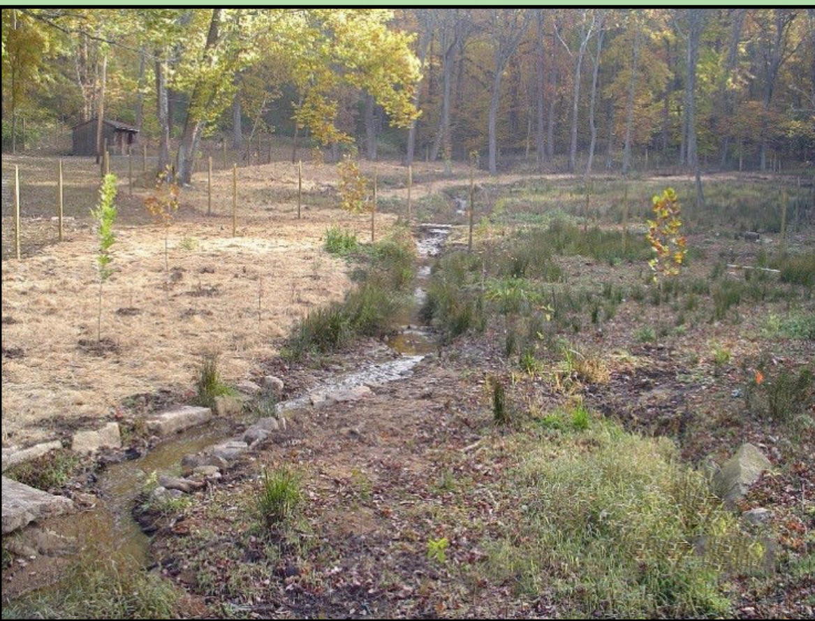
Post restoration photograph. Restoration included planting native trees, shrubs, and herbaceous plugs throughout the wetland area and modifying the stream channel to create more sinuosity, create aquatic habitat, and stabilize the stream banks.
