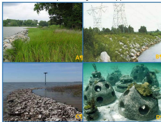
Figure 1: Example Living Shorelines Projects (A - Marsh Silt, B - Joint Planted Revetment, C - Oyster Reef, D - Reef Balls)
