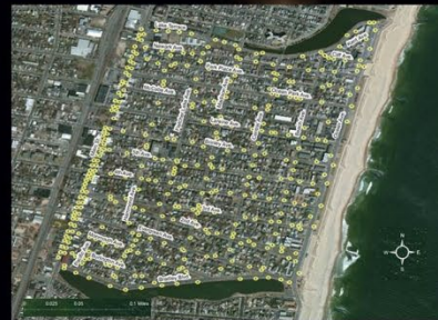
Figure 1: Aerial footage of Bradley Beach, NJ. Overlay displays each streetlight in Bradley Beach, along with the approximated area illuminated by each light.
