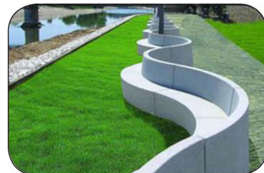
Example of Bench Floodwall
