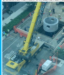
STORMWATER TREATMENT MANHOLE INSTALLATION
