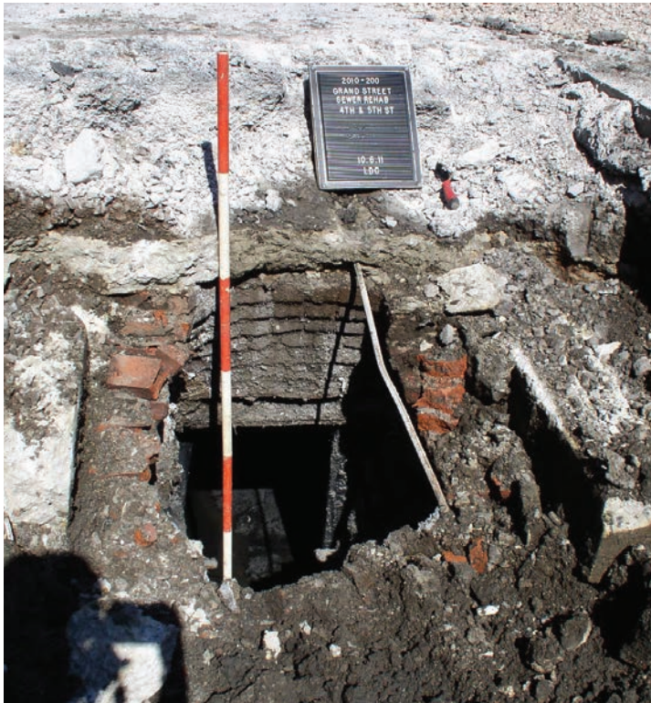
Photograph ES.4 Hoboken sewer monitoring with brick riser manhole
