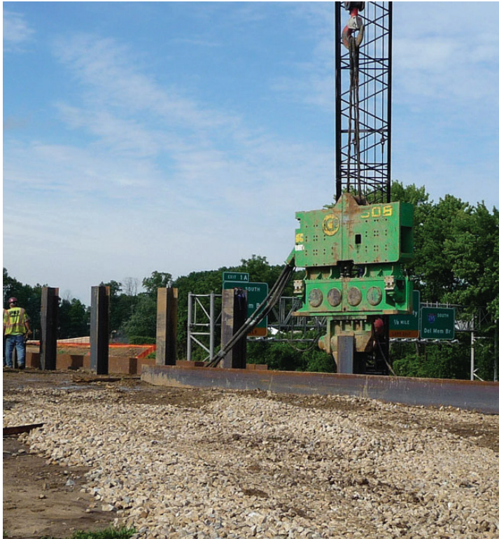
Photograph ES.3 Vibratory hammer - typical pile driving activity
