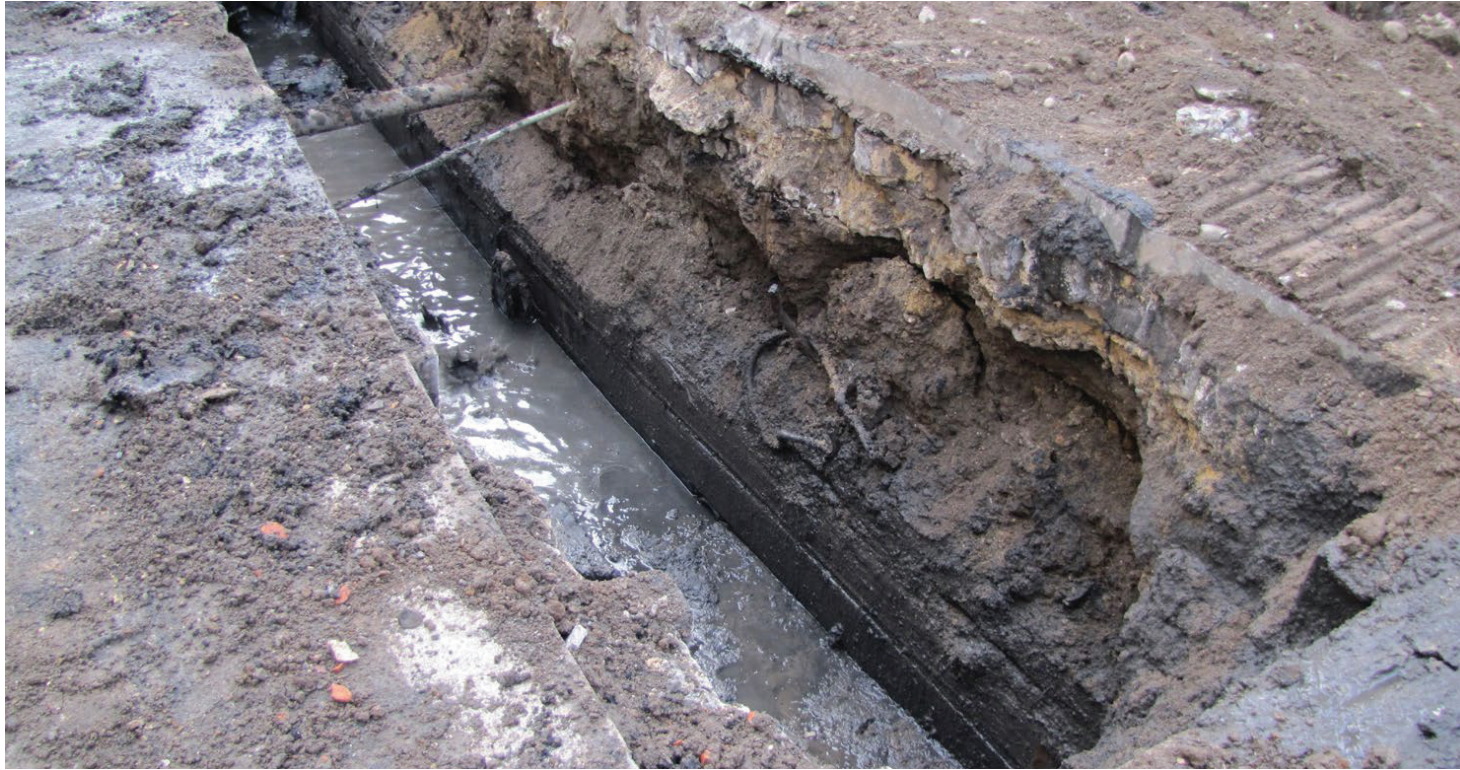
Photograph 4.8 Exposed Wood sewer, RGA 2015
